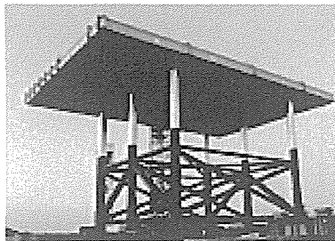
Prefabricated 30m high jacket unit
