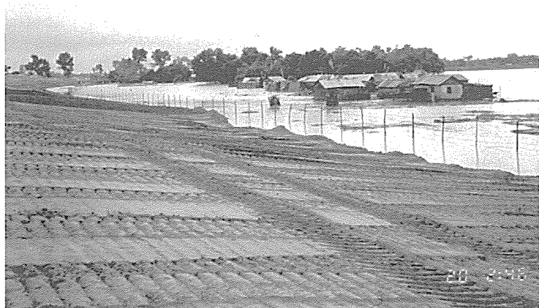
Sand slope behind the abutment zone
