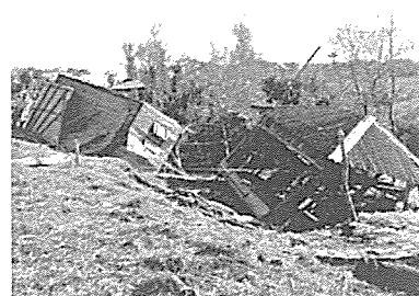
Small shops, businesses, and market areas were damaged along the road side
