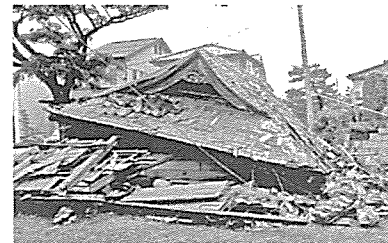
Old wooden structures collapsed at Kashiwazaki city
