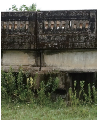
(a) The girder moved from the pier
