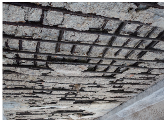
Photo 1: Damage to Thakhut bridge (Yangon)
