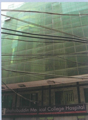
Educational institution with inadequate fire fighting system
