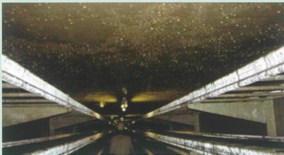
View inside box culvert structure
