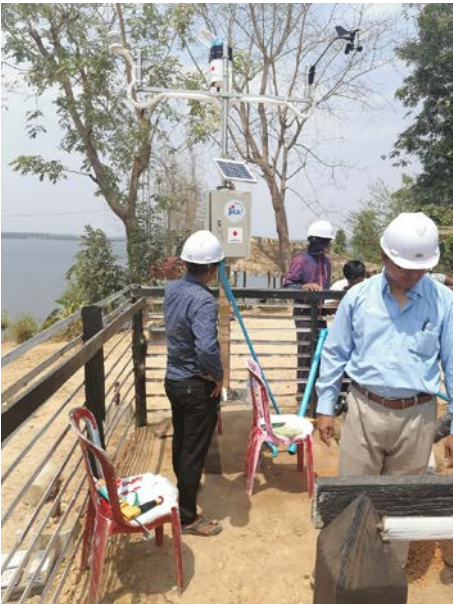
Installation of telemetry weather station and soil moisture sensor at Ma Zin Dam
