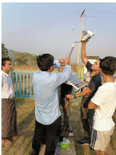
Re-installation of weather sensor at Tarwa Sluice Gate
