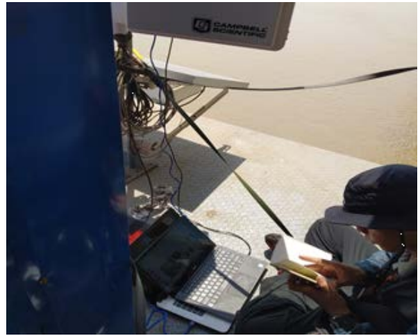
Maintenance of AHS at Dagon Bridge
