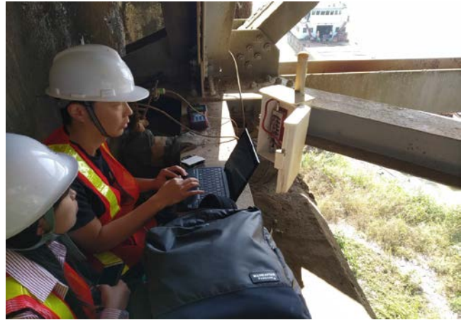
Data collection from inclinometer and Displacement Transducer
