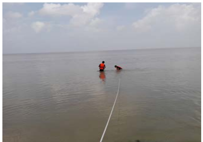
Installation of pressure sensor in the river before coming tidal bore
