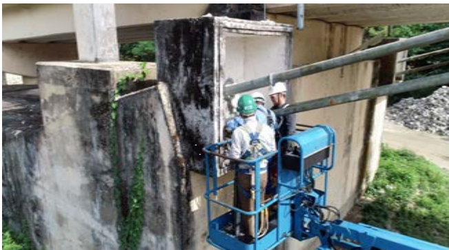
Inspection of anchorage condition in Shwe Laung Bridge
