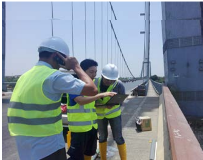
Explaining about the installation of the inclinometer
