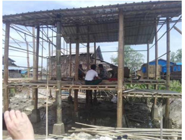
Observing the construction of new bamboo house at the slum area
