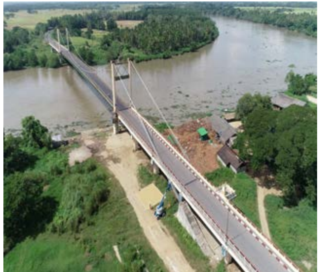
Overview of Panmawady Bridge and working area
