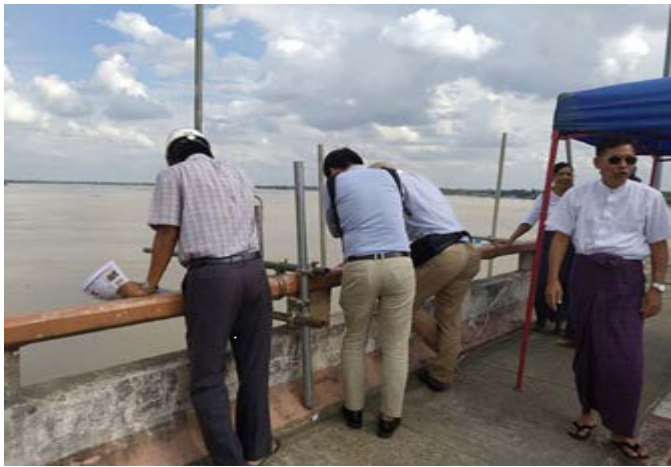
Checking the progress of construction of Automatic waterLevel Station at Kakawe Bridge
