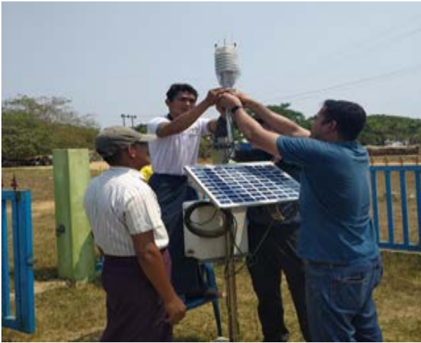
Maintenance of AWS at Tarwa Sluice Gate
