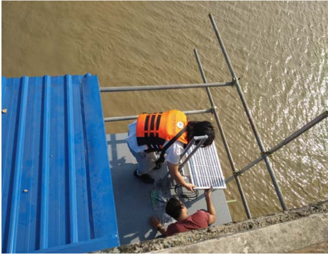
Preparation for the setting of solar panel
