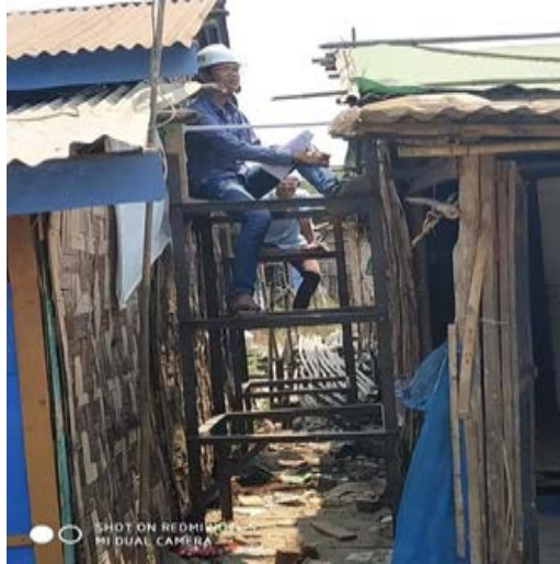
Pull-down test experiment in slum area of Yangon
