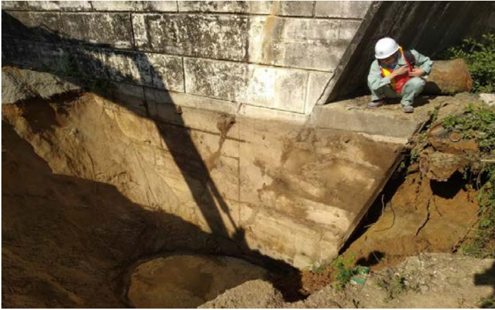
Excavation work to check the pile cap condition
