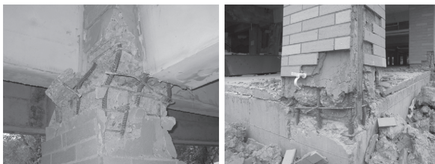
Photo 7: Flexural compression failure at the top and bottom of columns
