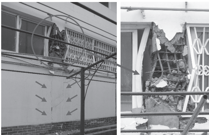
Photo 5: Shear failure in RC column shortened by partial height brick wall
