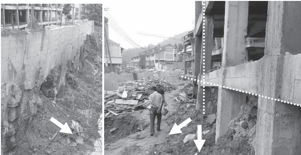
Photo 9: Structural damage due to soil failure
