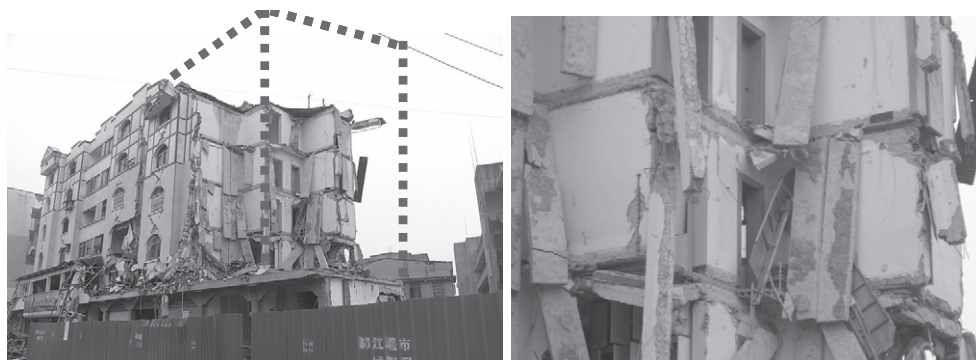
Photo 2: Partially collapsed brick buildings with hollow-core slabs
