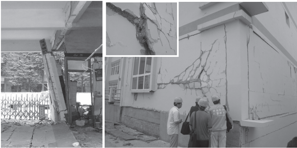
Photo 3: Shear failure in brick wall (left) and survived wall (right)
