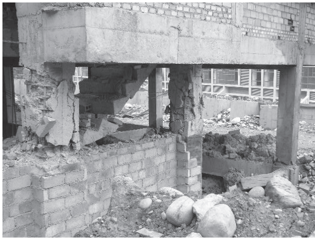
Photo 4: Typical shear failure in RC short columns
