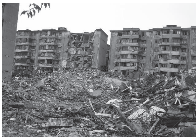
Photo 1: Seriously damaged brick buildings
