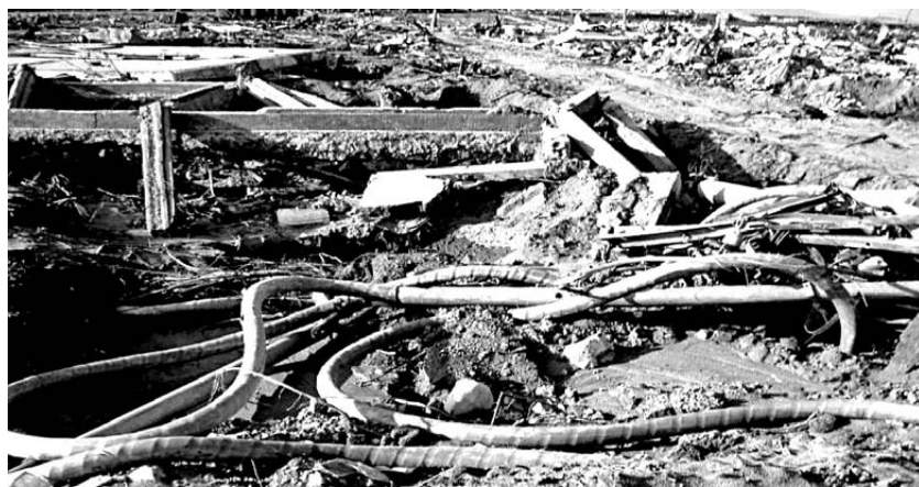
Electric cables poles toppled by battering, underground cables damaged by scouring and substation inundated
