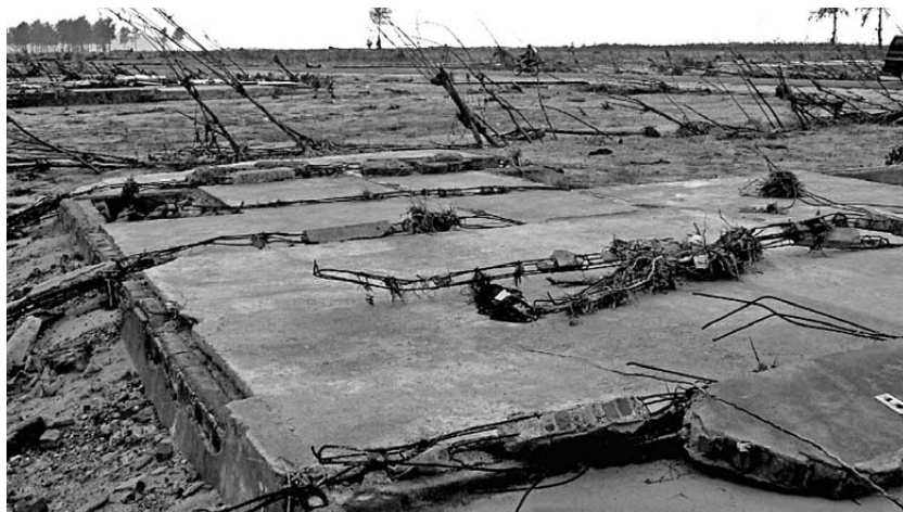
The poor detailing: a major cause of damage
