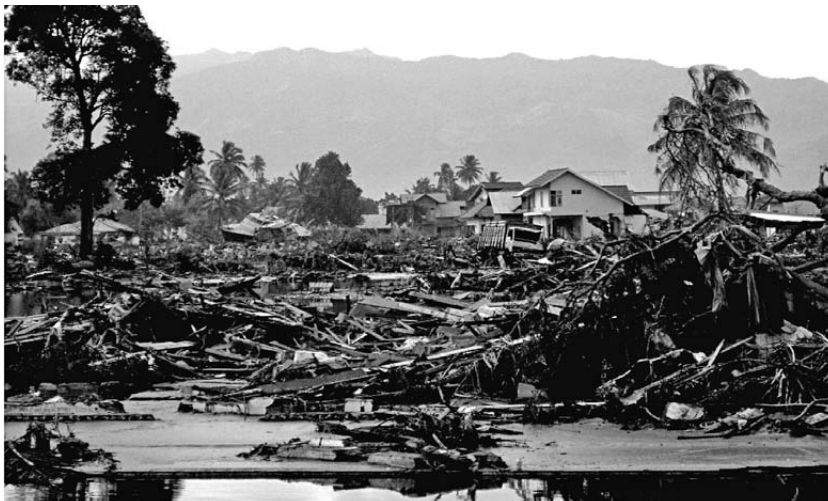
Banda Aceh: Zone 1; buildings damaged by battering and impact
