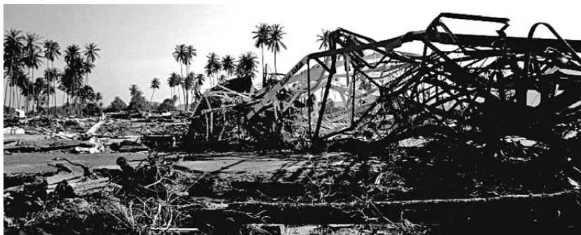
Telecommunication antennas swept by battering and dragged as far as 500 m
