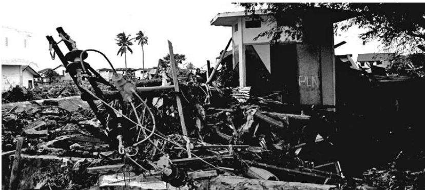
Electric cables poles toppled by battering, underground cables damaged by scouring and substation inundated
