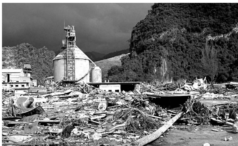
Cement Factory, Lhok Nga, damaged by battering, impact and buoyancy
