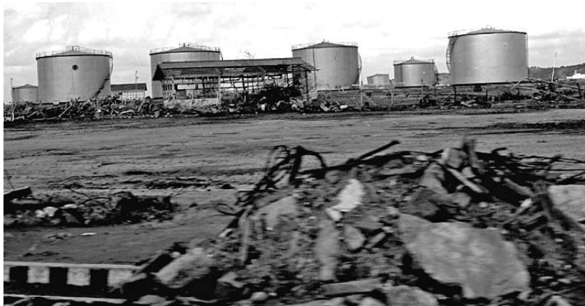
Cement Factory, Lhok Nga, damaged by battering, impact and buoyancy
