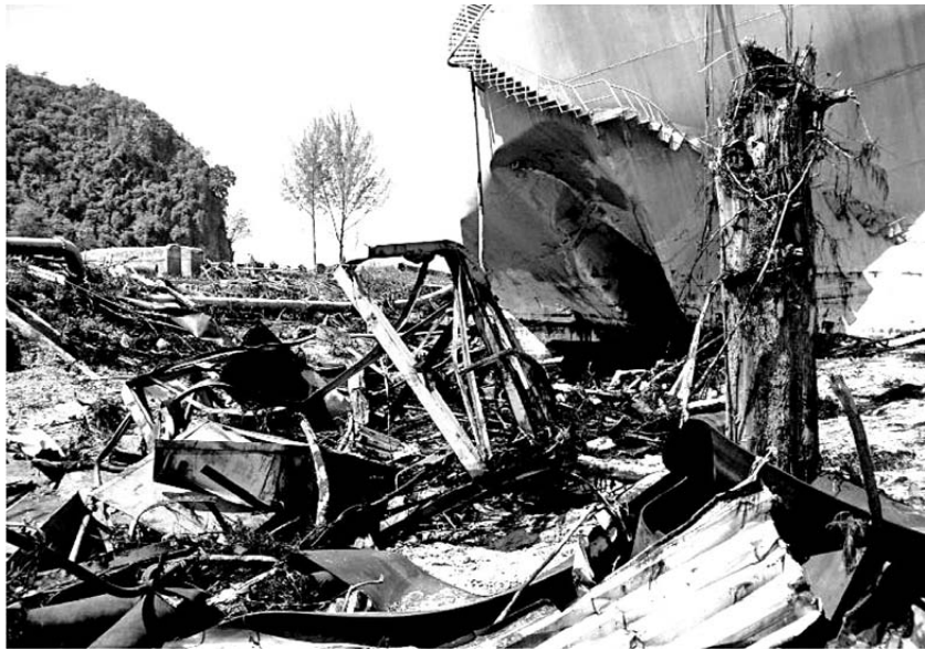
Cement Factory, Lhok Nga, damaged by battering, impact and buoyancy
