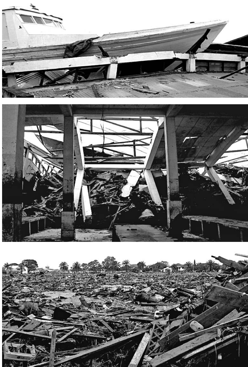
Banda Aceh: Zone 1; Buildings damaged by battering and impact
