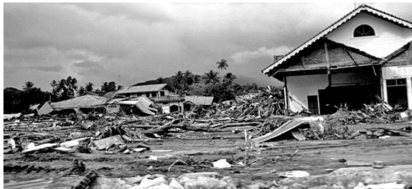
In Lhok Nga: Zone 1; Damaged by battering / impact
