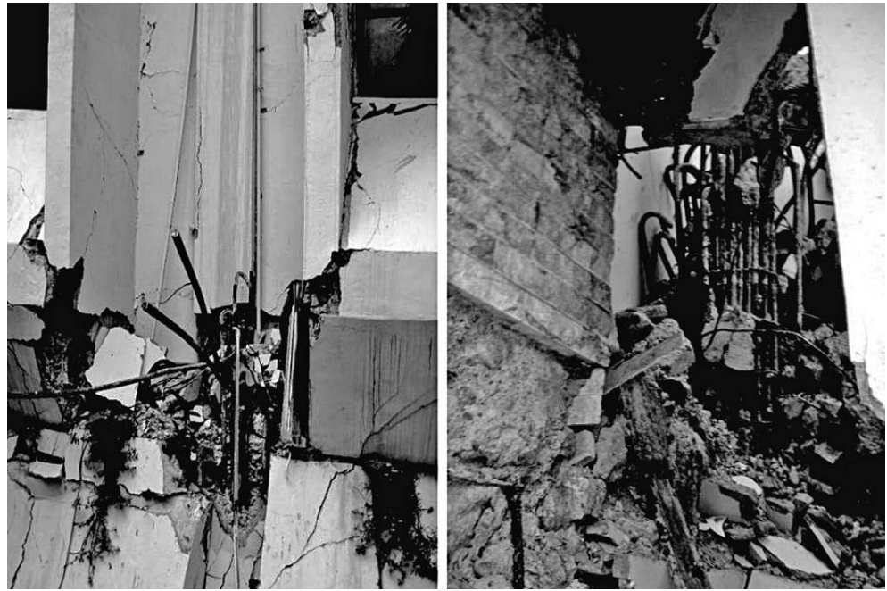
Exposed reinforcement after structural damage of Kuala Tripa Hotel
