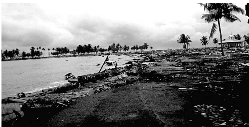
Meulaboh – Roads along the Coast damaged by Scouring
