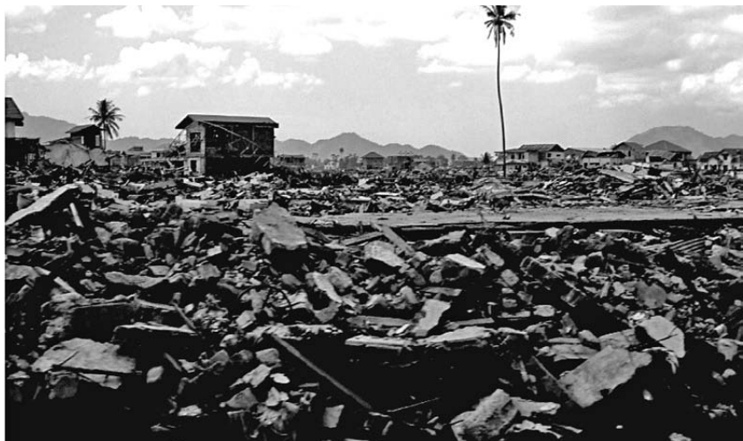
In Uluhe Lhe: Zone 1; Building damage by battering/ impact
