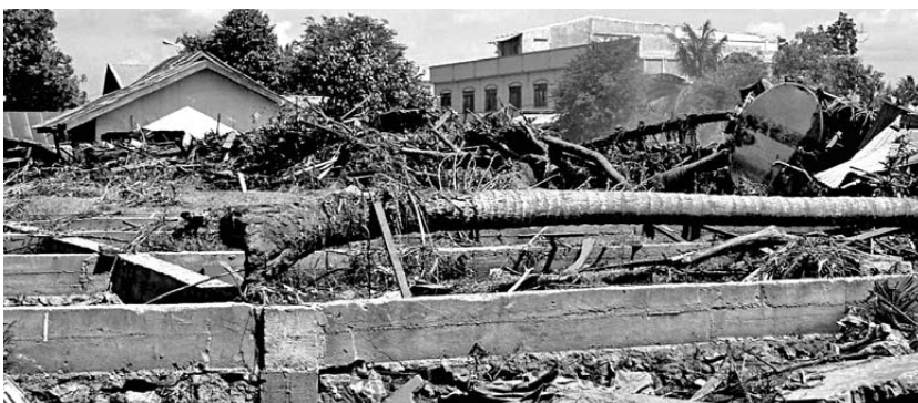
Banda Aceh: Zone 1; Building foundation scoured by tsunami
