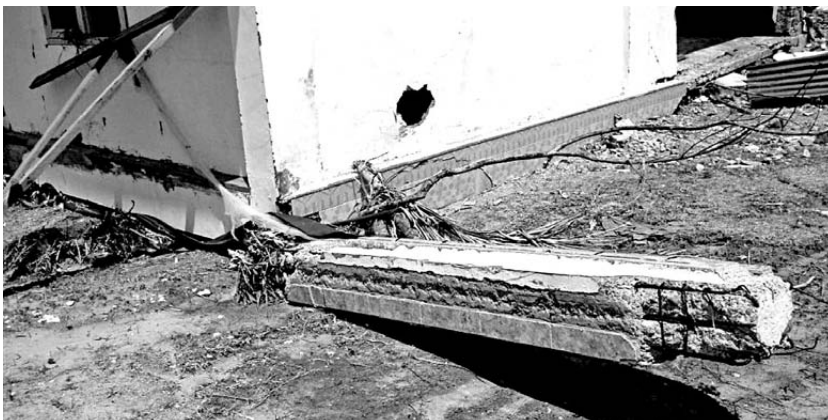
Unbelievable damage mainly due to poor detailing
