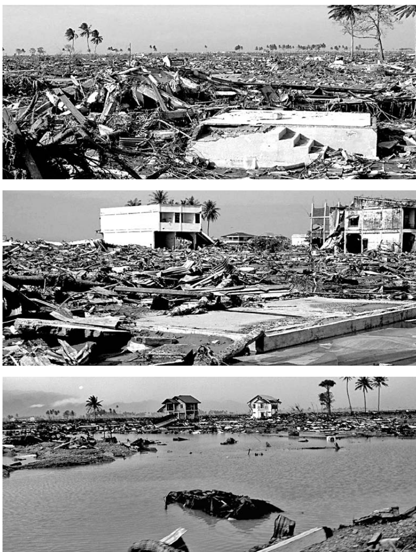
Banda Aceh: Zone 1; Building damaged by battering and impact
