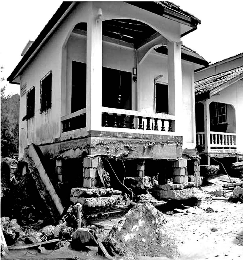
Figure 8: Floating foundations of a building in Phuket
