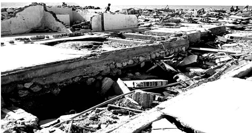
In Uluhe Lhe: Zone 1; Foundation scoured by tsunami
