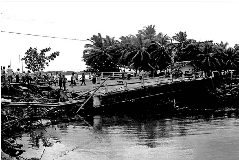
Figure 6: Almost all the bridges along the coast line water course have been damaged by the Tsunami. Temporary works have been done and the bridges made passable within a few days by the government organizations. (Source: CNO)
