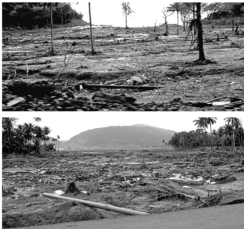
Water pipes unearthed and severed
