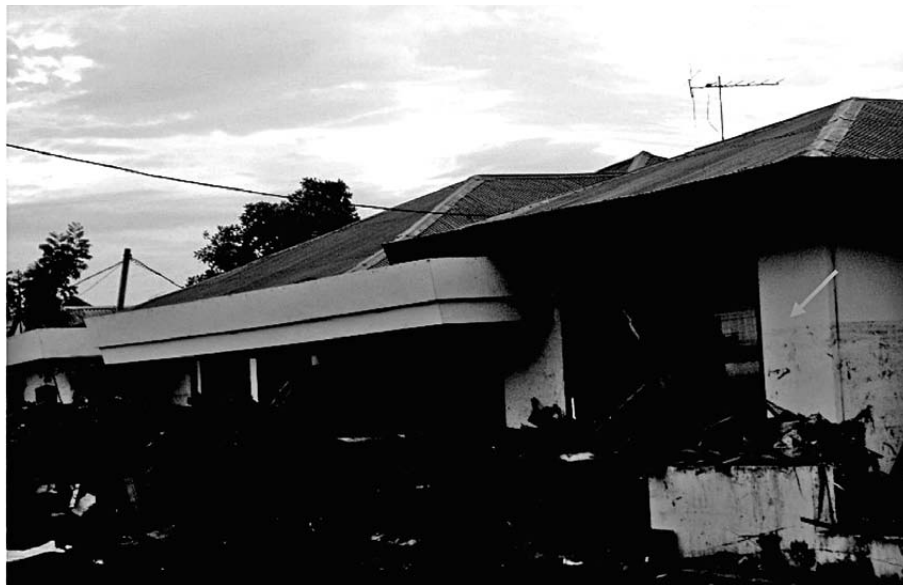
Inundation height observed in walls of a one story building in Banda Aceh
