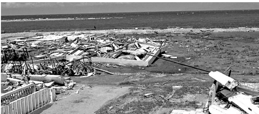
In Uluhe Lhe: Zone 1; Building damaged by battering/ impact
