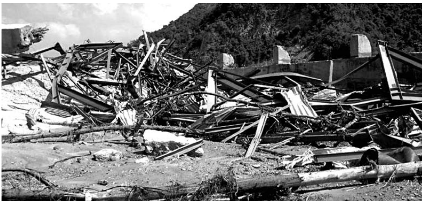
Cement Factory, Lhok Nga, damaged by battering, impact and buoyancy
