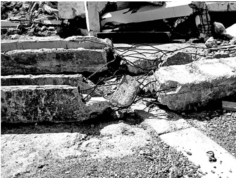
Poor detailing of buildings caused its structural damages into pieces
