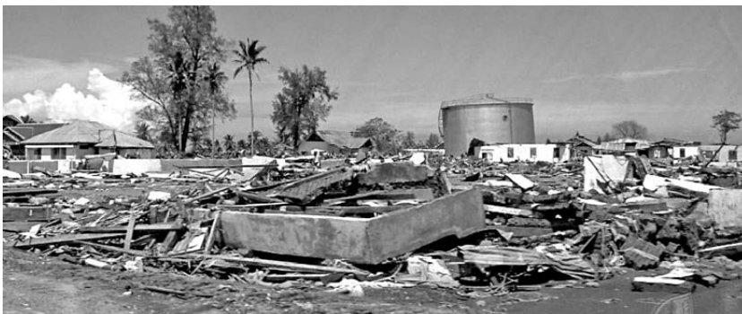
Krueng Raya: Zone1; Oil depot tanks dragged by floating / buoyancy
