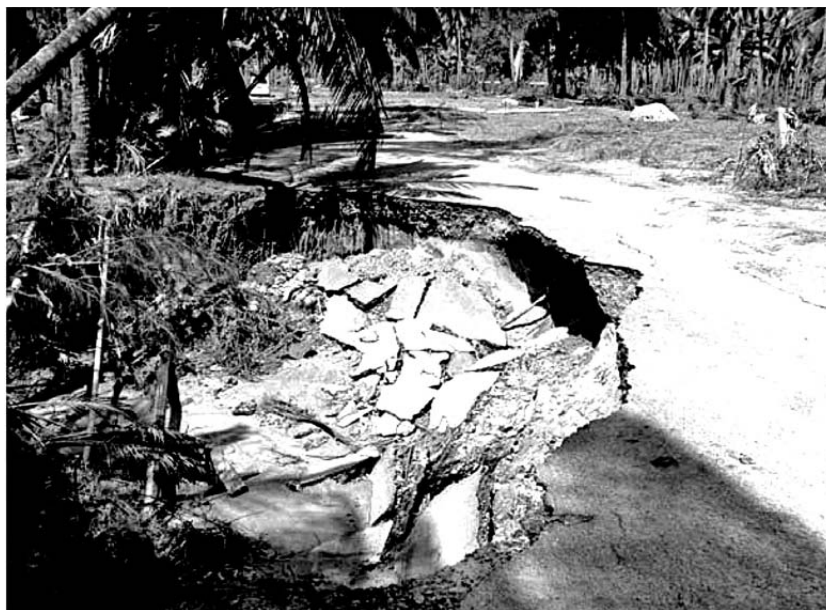
Figure 9: Severe scouring of road in Kuk-kak Beach
