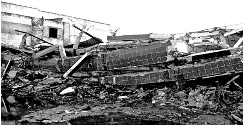
Damage due to poor detailing
