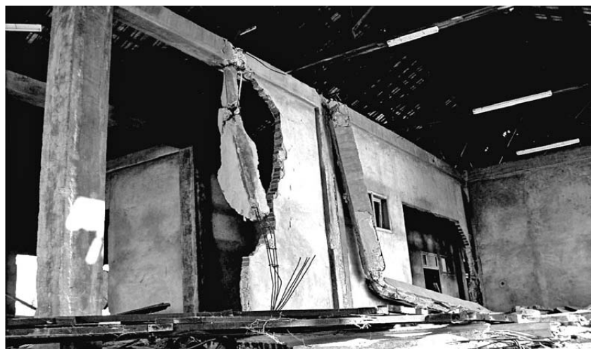
Damage due to poor detailing
