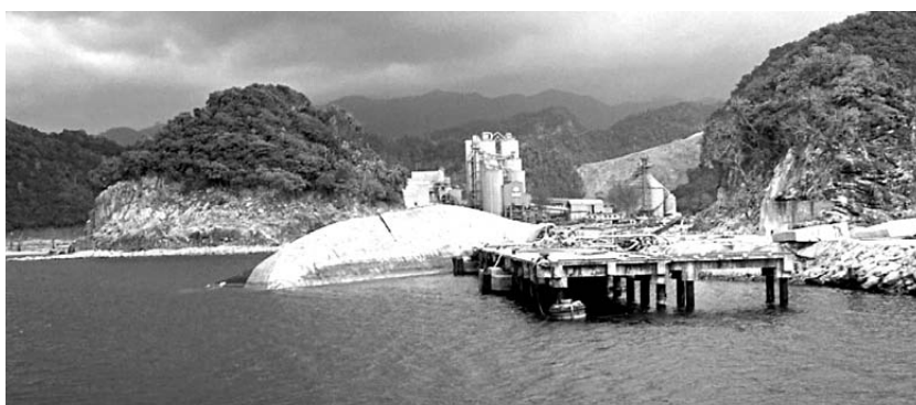
Lhok Nga Cement Factory Jetty is intact; slightly damaged by impact of boat
