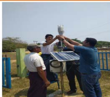
Maintenance of AWS at Tarwa Sluice Gate
