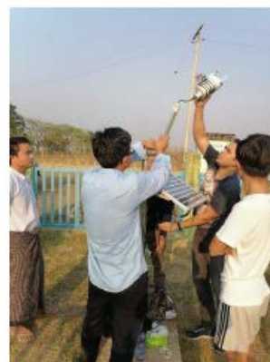
Reinstatlation of weather sensor at Tarwa Sluice Gate
