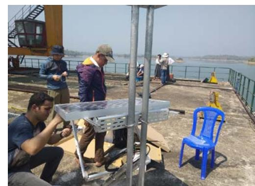
Preparation to install Automatic Hydrologic Station (AHS) at Zaung Tu Dam
