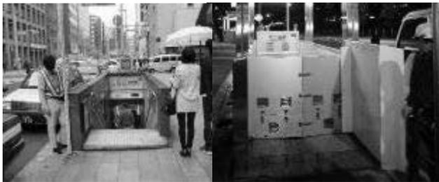
**Figure 5:** Bi-fold water stop door
