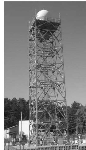
**Figure 8:** New Doppler radar used the train operation control against wind gusts
