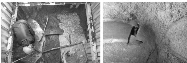
**Figure 1:** Photos of under cavities; left/ground water and joint failure of sewer, right/ broken sewer joint by aging
