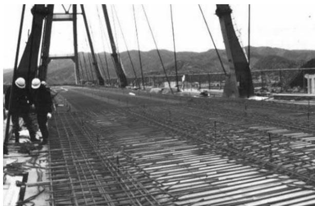
Figure 1: Epoxy-coated steel bars used for the reinforcement of concrete slab
