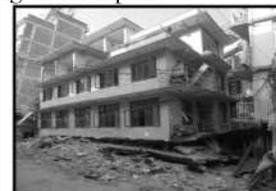
**Figure 2:** Soft storey damage of RC frame Building with open ground floor
