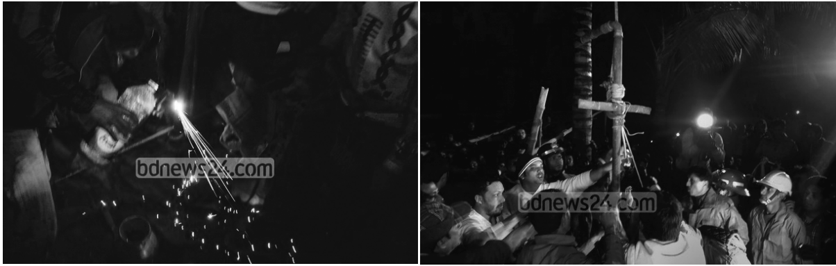
Figure: Uprooting of internal pipe
