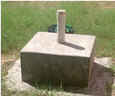
Figure 1: PVC pipe cased borehole.
