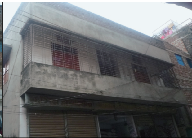
Figure 12: Heavy overhang of building
