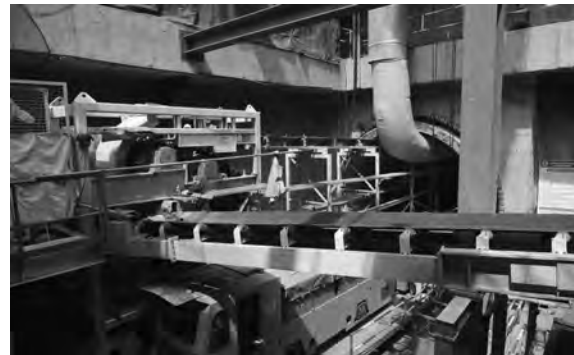
Process of excavating from the main tunnel
