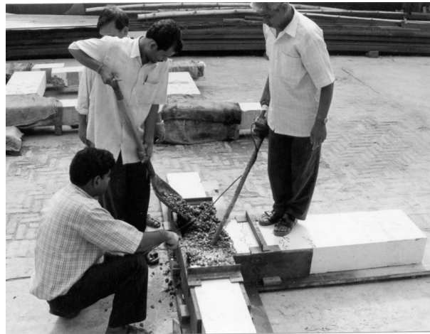
Figure 4: Putting fresh concrete after the removal of cracked concrete from failed joint
