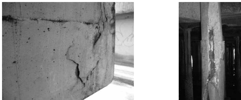
Figure 8: Concrete spalling due to carbonation induced steel corrosion in Bangkok area (left) and chloride induced corrosion in eastern part of Thailand (right) (Maintenance problem)
