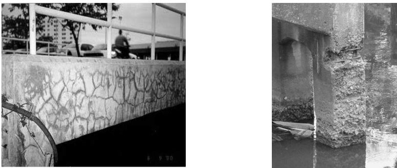
a) Cracks due to AAR
