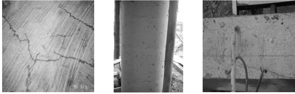
Figure 6: Plastic shrinkage (left) and plastic settlement cracking (center and right) showing construction problems
