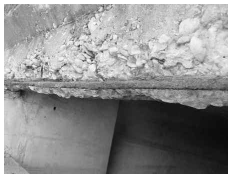
Figure 5: Severe honeycombing due to segregation (Problem of concrete mix proportion)
