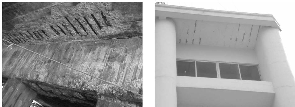
Figure 7: Steel corrosion due to insufficient concrete cover under a bridge (left) and in a building (right) (Construction problem)
