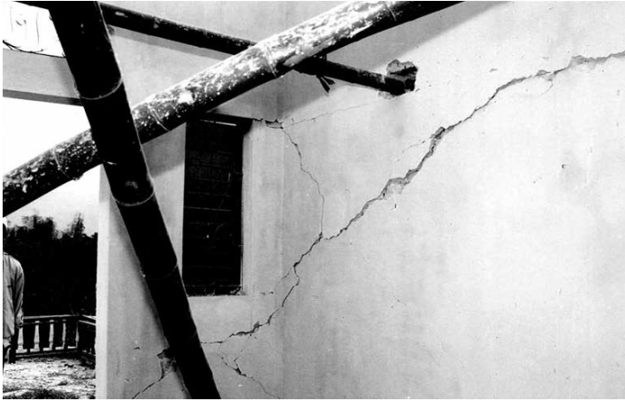
Figure 1: Damage of bearing wall
