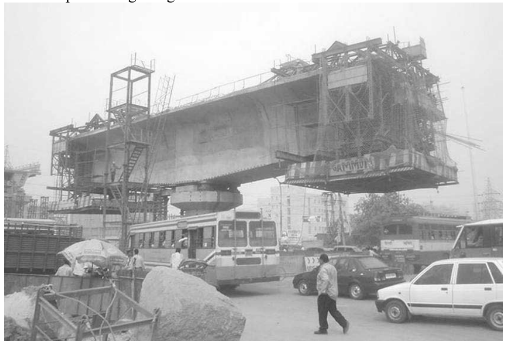
Figure 2: Pitampura Cantilever Bridge no disturbance to Traffic (38.5m + 55m + 38.5m)
