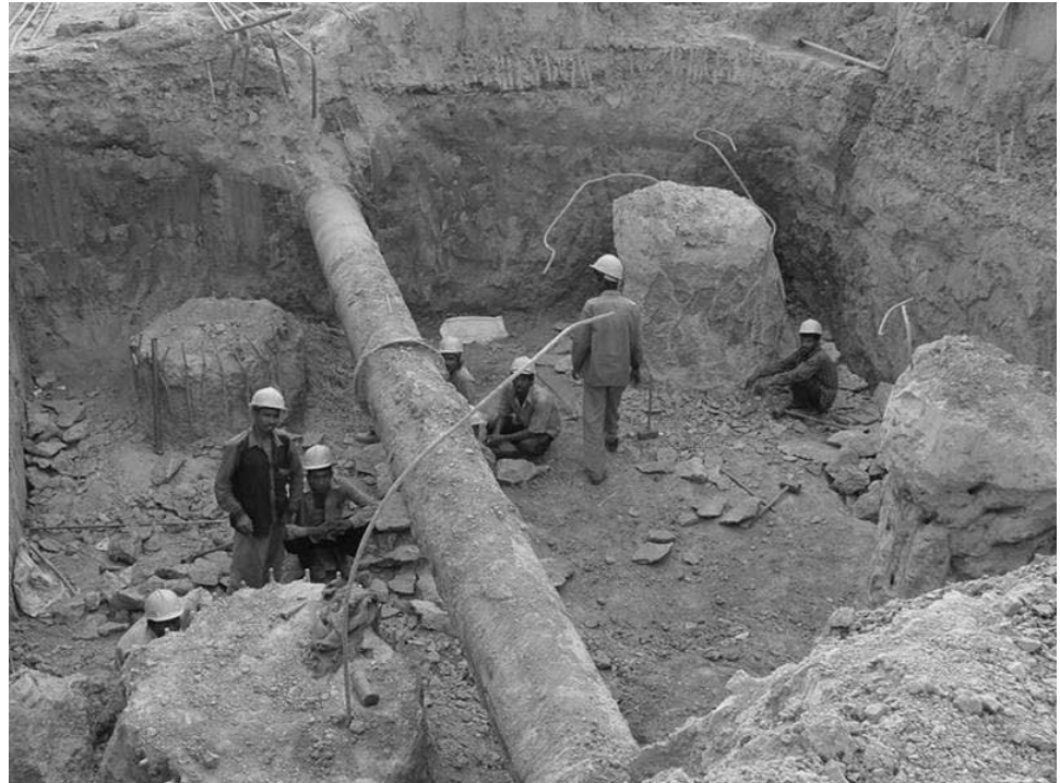
Figure 8: Irregular Configuration of Piles for Straddling Across
