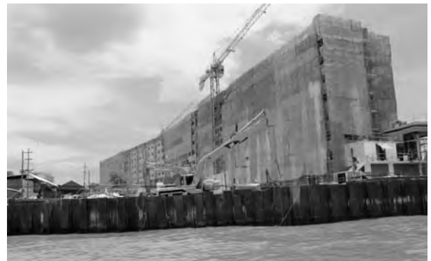
constructing a flood wall with concrete beams and slabs
