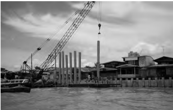
constructing a flood wall with concrete beams and slabs
