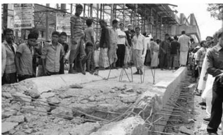
The girder which collapsed at 29 June, 2012
