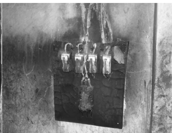
Figure 8: Burnt electric switch board
