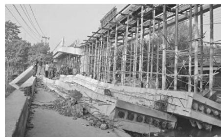
The girder which collapsed at 24 November, 2012
