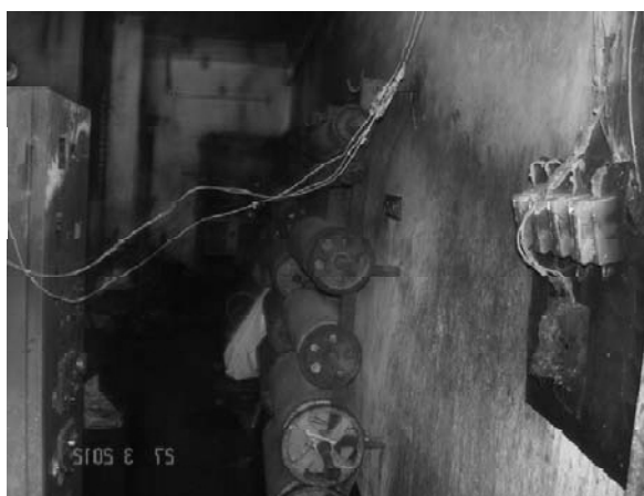
Figure 7: Burnt wire and electric switch board
