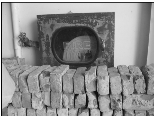
Photograph 7: Blocked hose pipe
