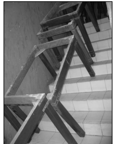
Photograph 12: Blocked emergency stair case in a commercial building
