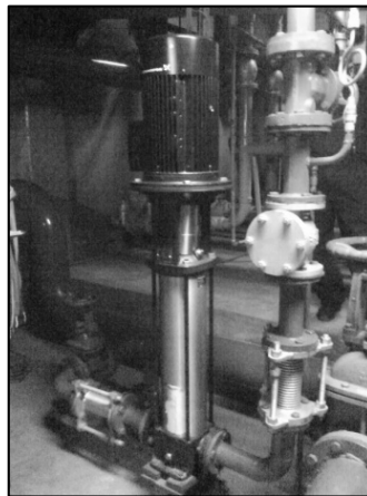
Photograph 5: Jockey pump in commercial building
