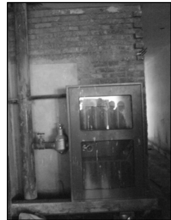
Photograph 6: Hose reel with stand pipe in commercial building
