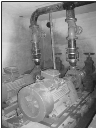
Photograph 4: Fire pump in commercial building
