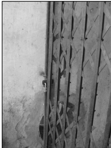
Photograph 12: Blocked emergency stair case in a commercial building
