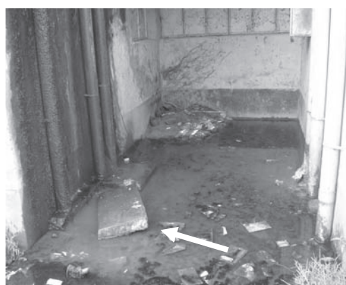
(e) Inactive Soak well due to over flow during rainy season
