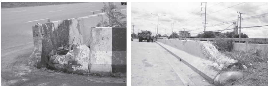
Figure 7: Untreated Barrier Ends
