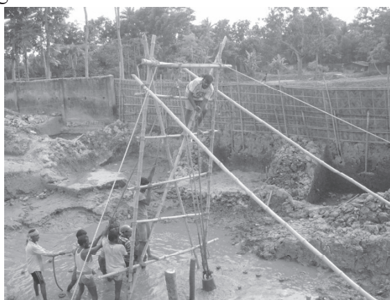
Figure 16: Picture of Timber Pile driving.
