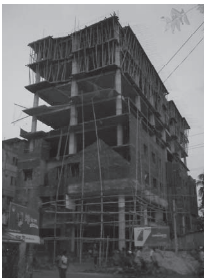
Figure 10: Construction picture of Nurgis memorial clinic Building
