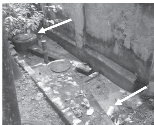
(a) Inactive soak well & direct discharge of Sewage into KCC drain
