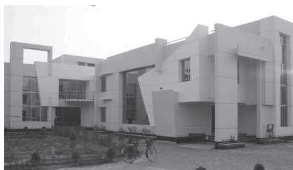
Figure 17: Pictorial view of AITI Administration Building
