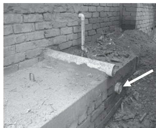
(b) Newly constructed building without soak well
