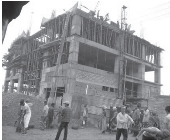
Figure 12: Construction picture of Delta Life Insurance Building
