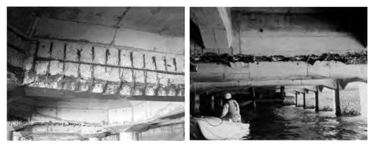
Figure 1. Examples of deterioration on reinforced concrete beams of open-type wharf
