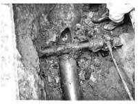
A water pipe broke an existing sewer pipe, found under a cave-in
