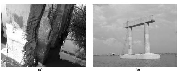
Fig. 13 Picture of actual inspected structure (a) Bad quality (b) Good quality.
