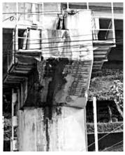
Corrosion of steel due to the use of sea sand as fine aggregate
