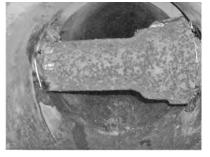
A water pipe passing through an existing sewer pipe, found under a cave-in
