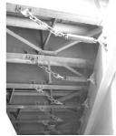
Apparatus to prevent the fall of bridge girders
