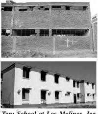
Top: School at Los Molinos, Ica. Note that columns in the 1st and 2nd floor are either not aligned or interrupted. Bottom: Hospital at Pisco, where 80% of the houses were affected, suffered no damage.
