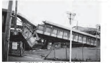
Collapsed RC bridge due to the 1995 Kobe Earthquake
