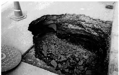
A cave-in due to failure of a corroded sewer pipe
