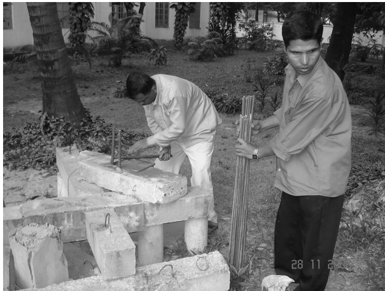
Figure 4: Bending of stirrups and tie rods.
