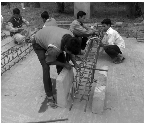
Figure 5: Beam and column preparation.
