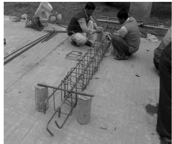
Figure 5: Beam and column preparation.
