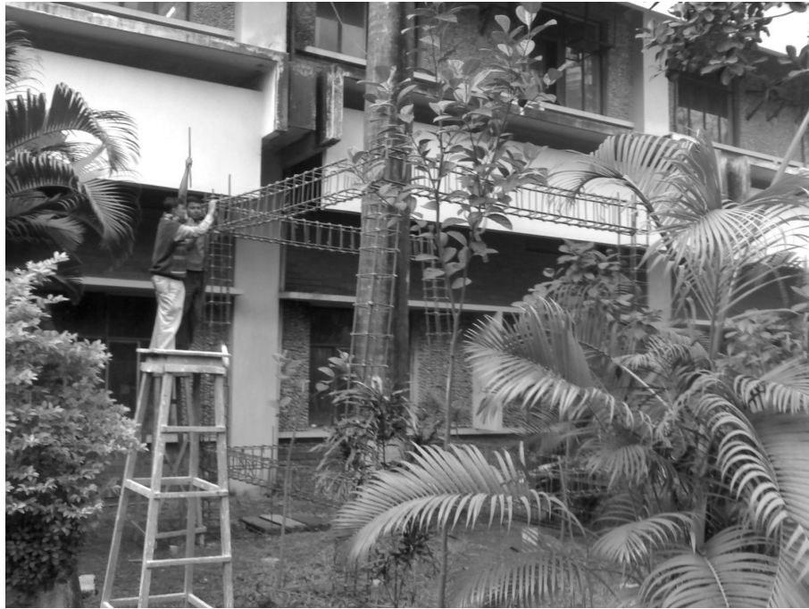
Figure 6: Beam and column fixing.
