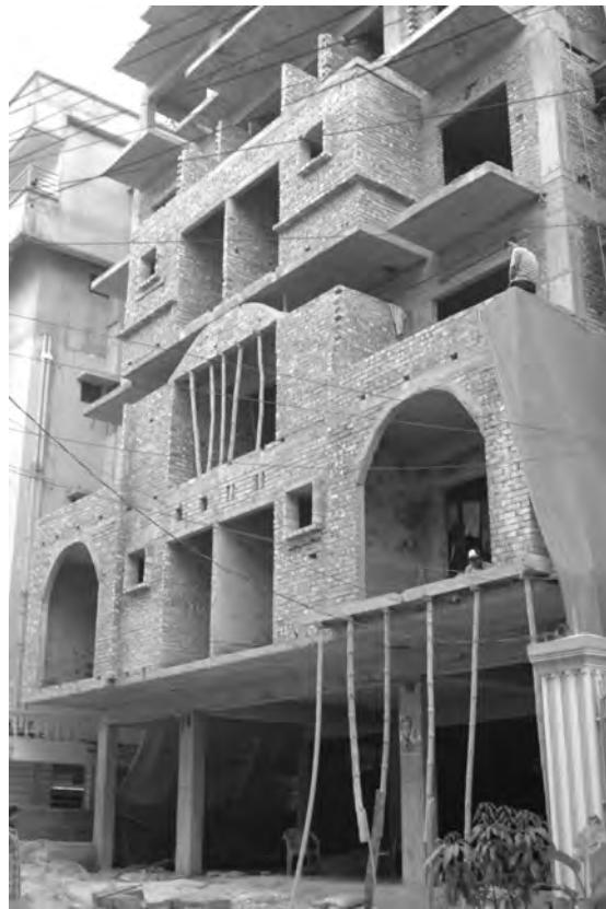
*Figure 20: Soft storey and heavily overhanging structure in Dhaka*
