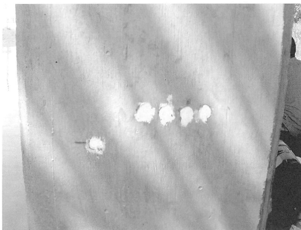
Figure 28: Epoxy filled hole after collecting the sample
