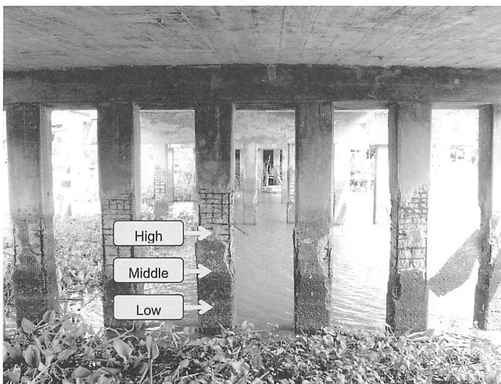
Figure 24: Location of collecting concrete powder sample
