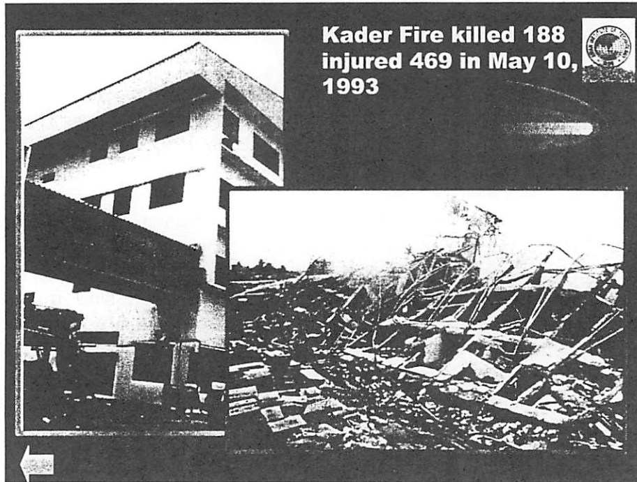
Figure 1: Fire in naked steel toy factory killing 188 in 1993.
