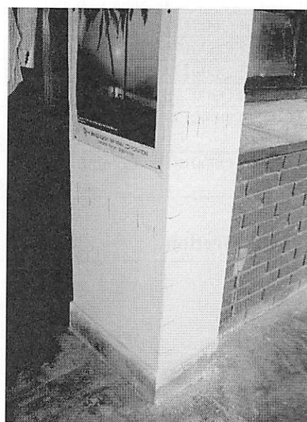
Figure 36(b) Marking of column reinforcement at the ground floor of Titumir hall.
