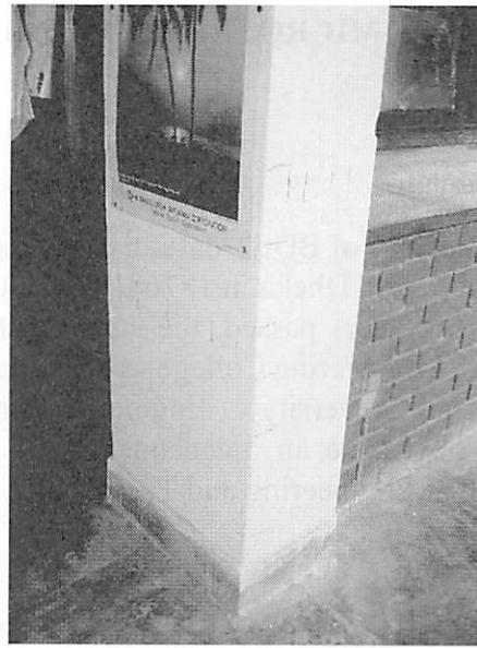
Figure 7(b) Marking of reinforcement in a column at ground floor of Titumir hall.
