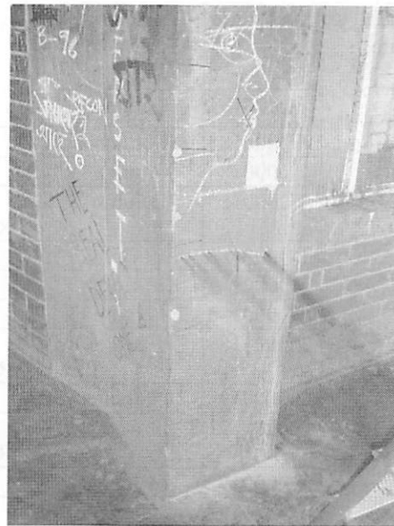
Figure 23(b) Marking of column reinforcement at the ground floor of Architecture building
