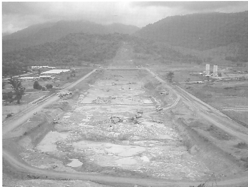
Figure 24: Foundation excavation of the main dam
