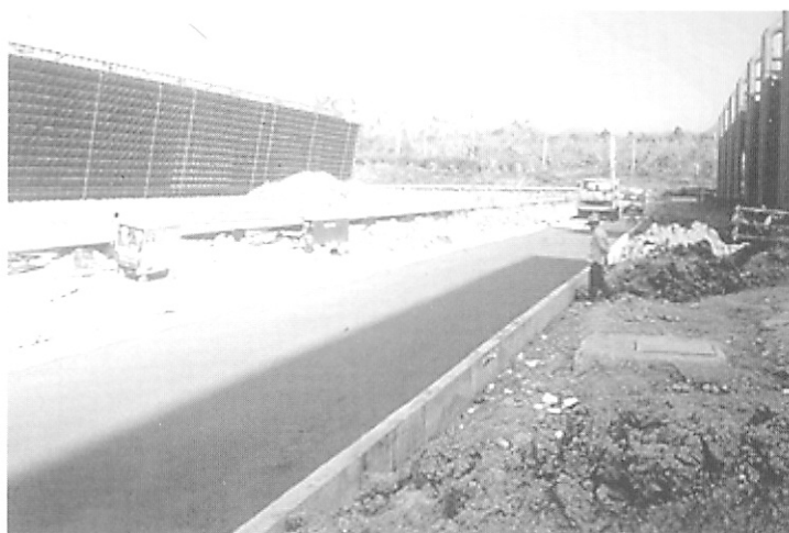
Figure 9: Demonstration construction of Roller-Compacted Concrete Pavement using fly ash at Mae Moh power generating plant
