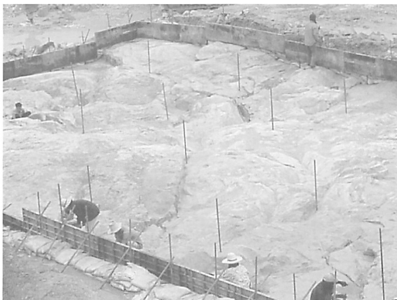
Figure 25: Rock foundation of the dam was clean and all weathering rock was removed before placing the leveling concrete
