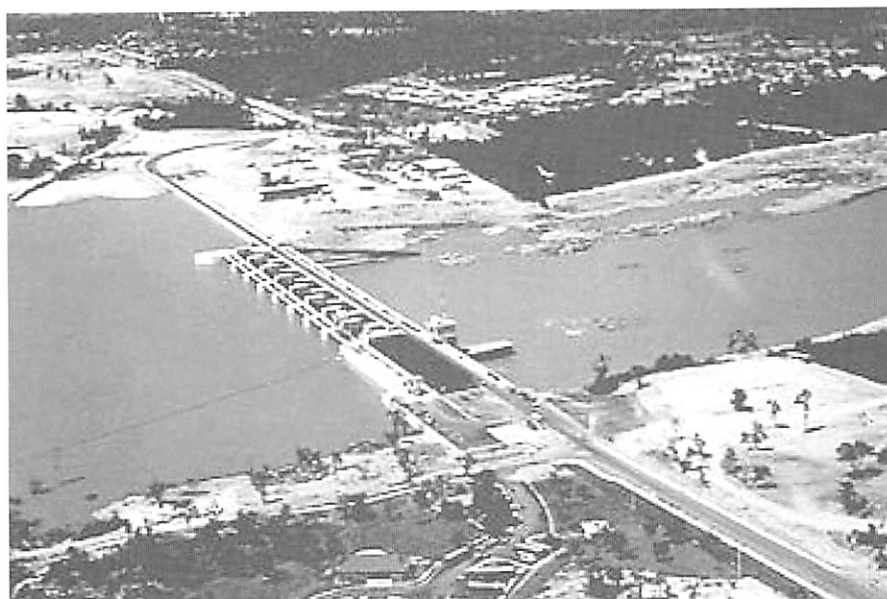
Figure 17: Pak Mool dam in Ubol Rachathani constructed using roller-compacted concrete with fly ash content of 68% of the total cementitious materials.
