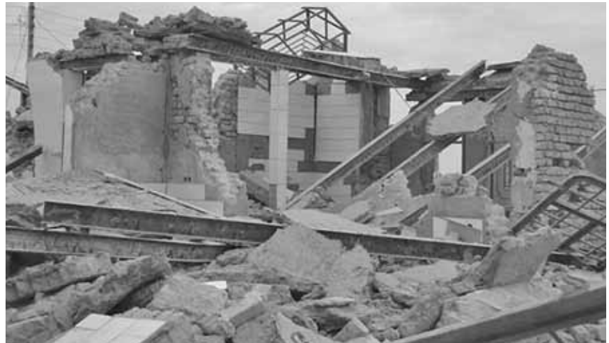
Failure of unreinforced masonry walls and collapse of roof beams
