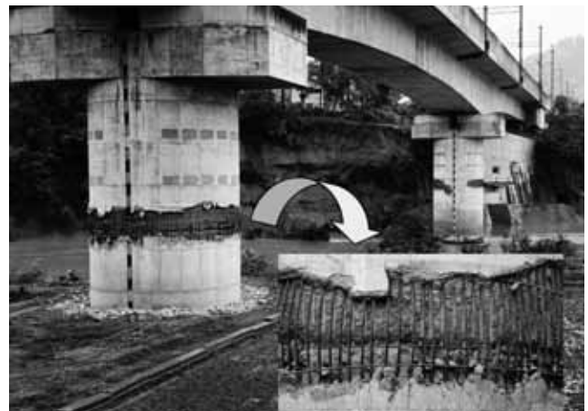
Bullet train viaduct pillars exhibited concrete spalling at the sections where longitudinal rebars were cut
