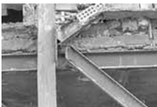
Separation of x-bracing elements from the column due to poor quality of welding
