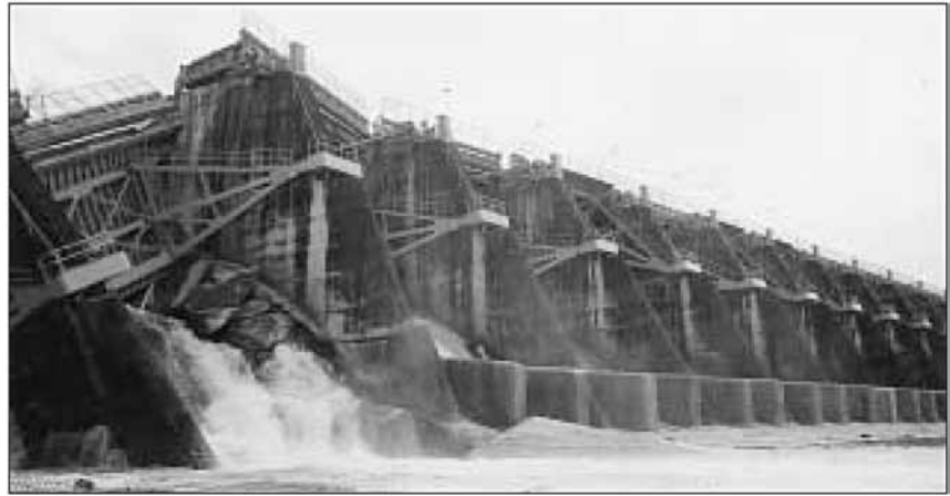
Shi-Kang water supply weir damaged during the Chi-Chi earthquake (Mw 7.5) of September 21, 1999 in Taiwan (courtesy: K. Meguro)
