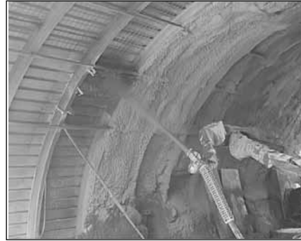
Shotcreting using automated equipment
