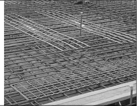
Use of FRP rods along with conventional steel reinforcement
