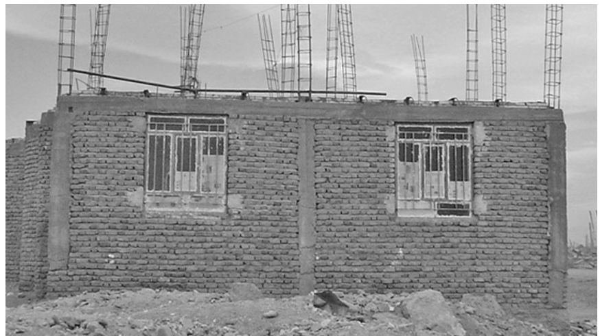
Vertical and horizontal ties maintain the stability of building
