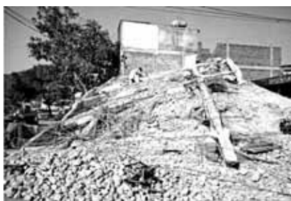
Pancake collapse of building (Abbottabad)
