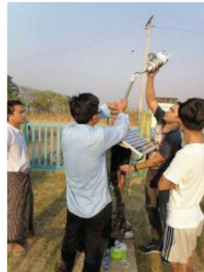
Reinstatllation of weather sensor at Tarwa Sluice Gate
