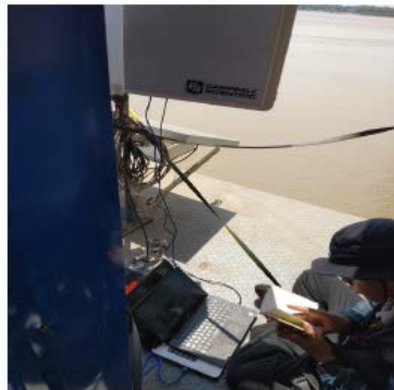
Maintenance of AHS at Dagon Bridge
