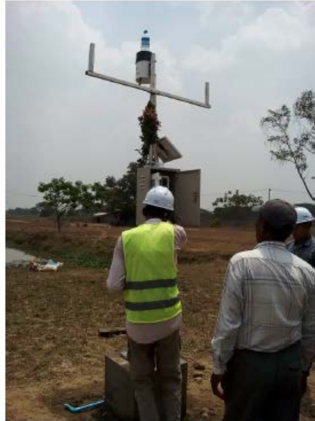
Installation of telemetry weather station at Shwe Hlay Sluice Gate
