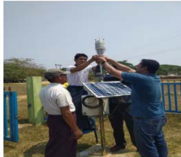
Maintenance of AWS at Tarwa Sluice Gate
