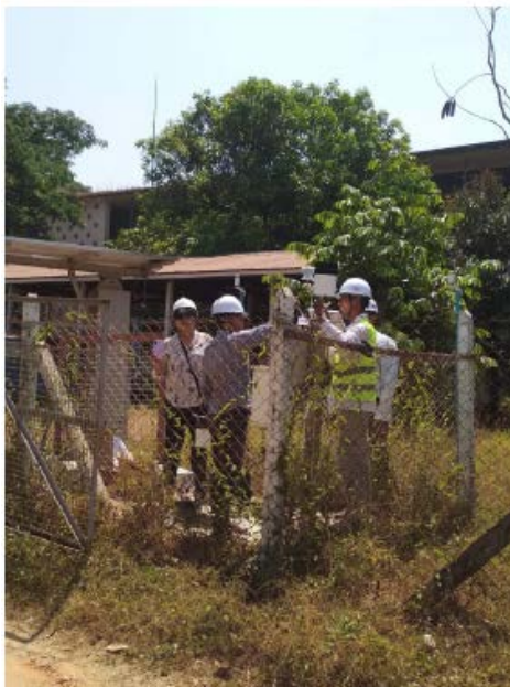
Installation of telemetry weather station in YTU campus
