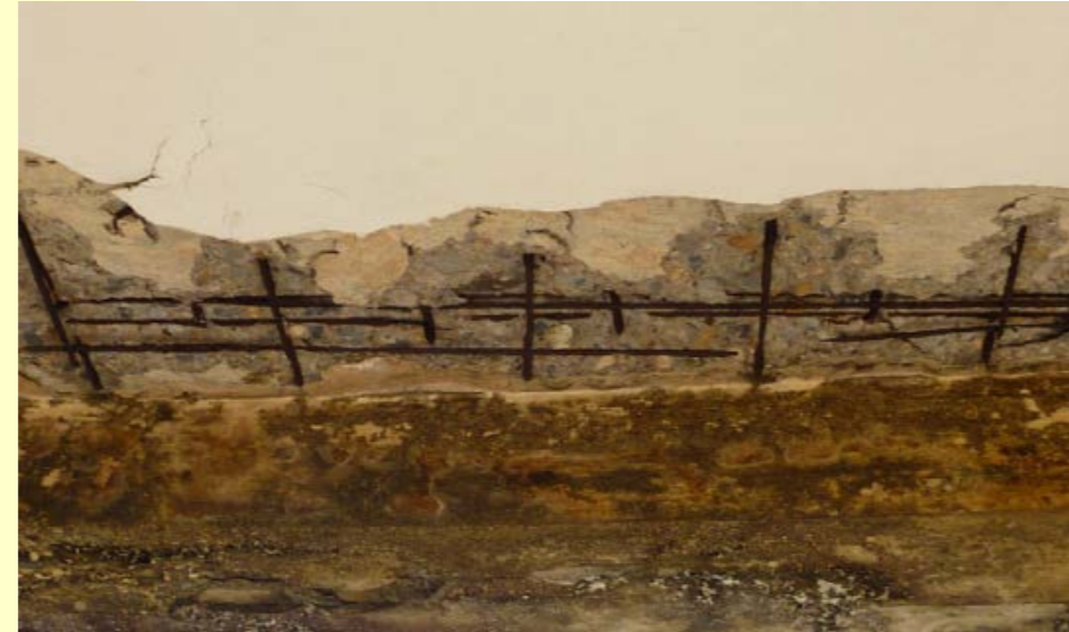
Inspection of concrete structures in Myanmar
