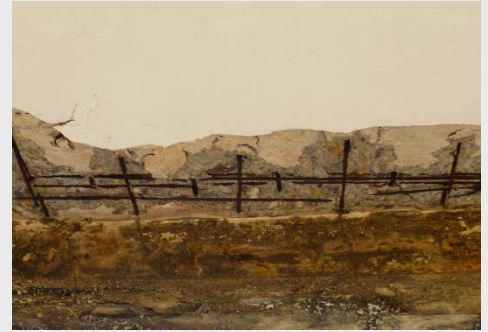
Inspection of concrete structures in Myanmar
