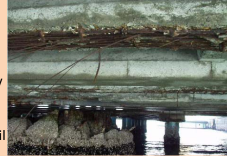
Chloride-induced deterioration of a structural concrete member
