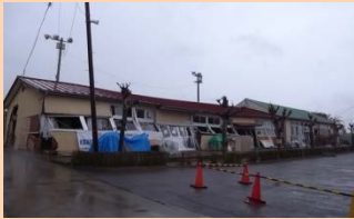
Damage survey of wooden houses caused by the 2011 Great East Japan Earthquake and Tsunami
