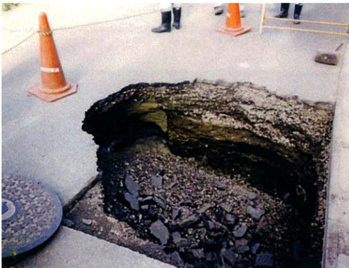
Cave-in due to the corrosion failure of sewer pipe
