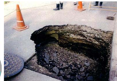
Image of sagging road by damaged sewage pipe
