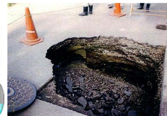
Image of Sagging Road by Collapsed Sewage Pipe
