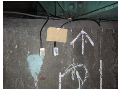
Bridge Vibration Measurement
