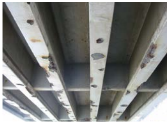
Degradation structure investigation
