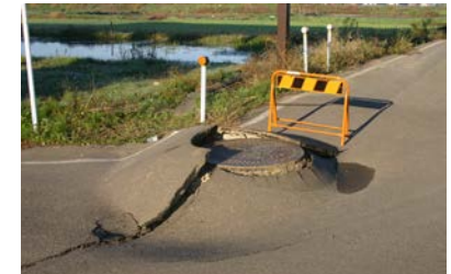
Earthquake disaster investigation
