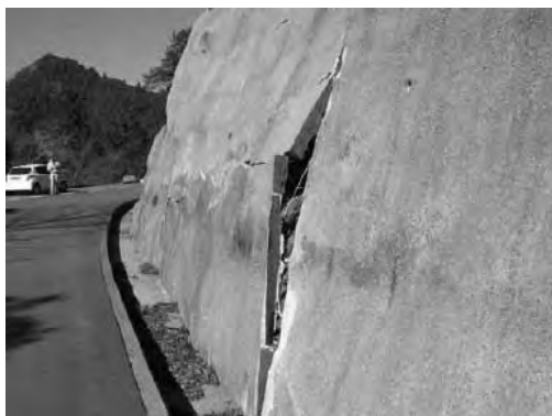
Figure 7: Degradation damage of the excavation slopes (Ministry of Land, Infrastructure and Transport website)
