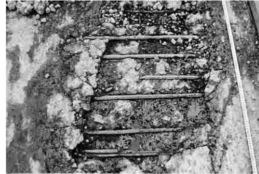
Figure 5: Degradation of road bridge floor board concrete
