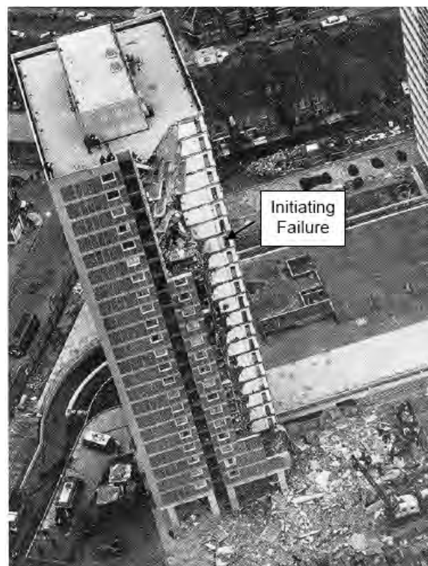
Figure 1: Ronan Point collapse: a gas explosion on the 18th floor resulted in a progressive collapse
