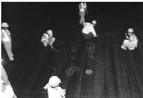
Figure 17: The hammering test by night inspector
