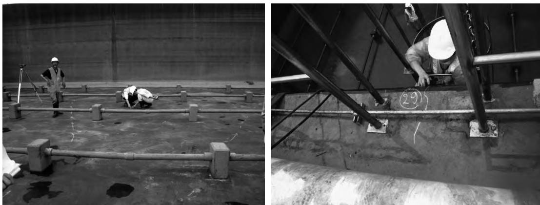
Figure 1: Cracks on Waste water pond (Thermal Power plant)
