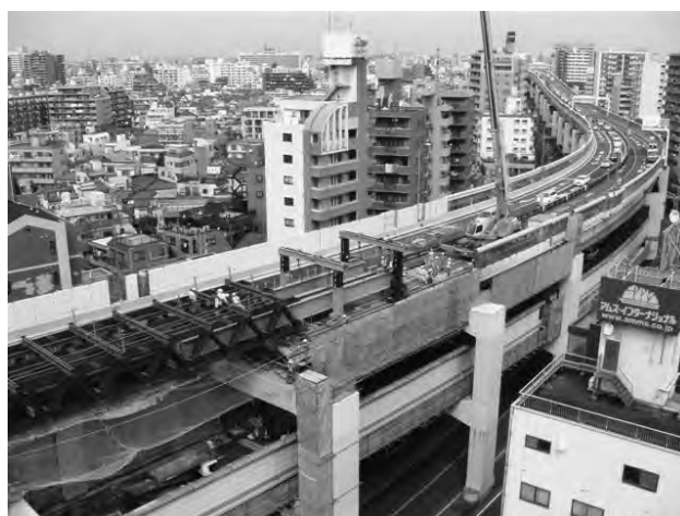
Photo 4: Restoration Work 1 (Removal of damaged girders)
