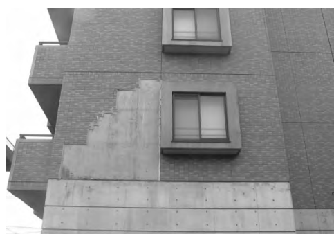
Figure 2: The case of tile detached itself
