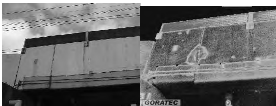
Figure 15: The float that occurred on the wall of the bridge railing
