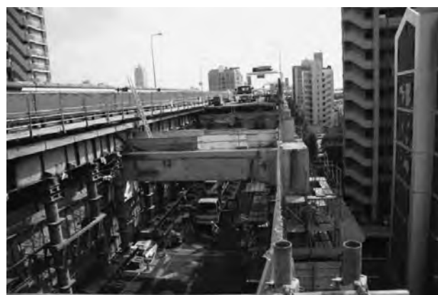
Photo 5: Restoration Work 2 (Setting of New Girders by the election girder)
