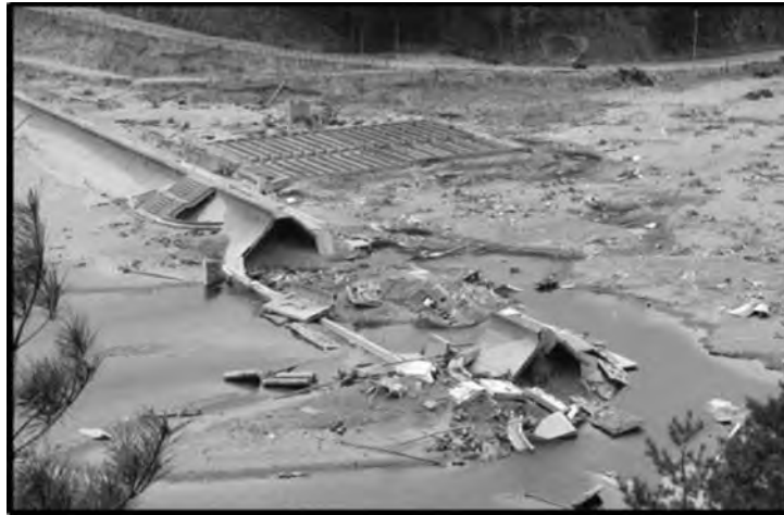
Figure 1. A typical fill-type coastal dike that fully collapsed by tsunami, Aketo, Tanohara, Iwate Prefecture (courtesy of Koseki, J., Univ. of Tokyo)
