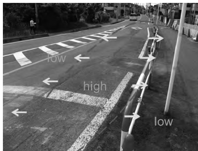
Figure 2: Significant ground settlement in the area
