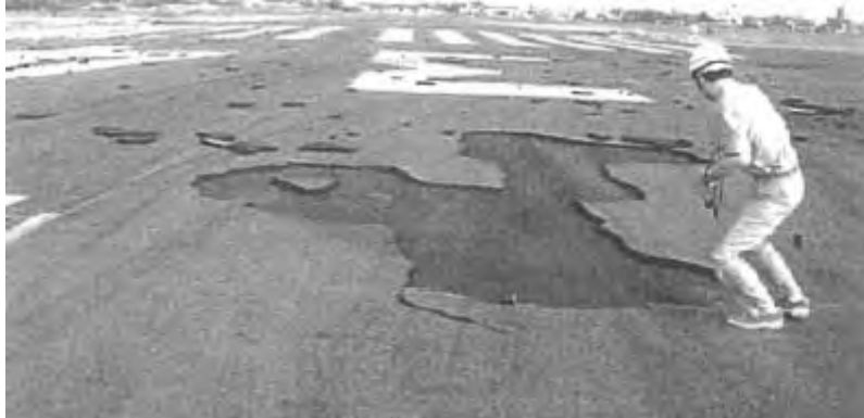
Figure 8: Pavement peeling of the airport runway ((Ministry of Land, Infrastructure and Transport website)
