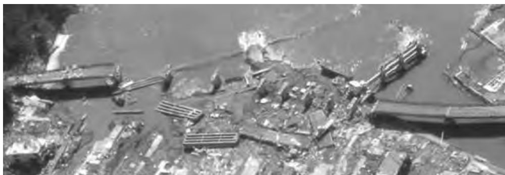
Figure 8: Bridge girders washed away from their piers by Tsunami (Photo: Tohoku Regional Bureau of MLIT)
