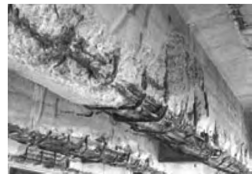
Figure 6: Degradation damage of road bridge main girder (Ministry of Land, Infrastructure and Transport website)
