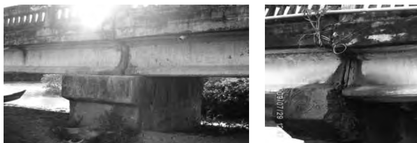
Photo 3: Displacements of beams at Thakyut Bridge
