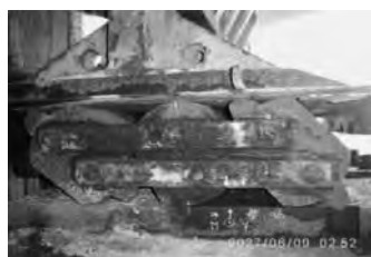
Photo 1: Deformed locker shoes on end pier Photo 2: Deformed shoe on pier 7
