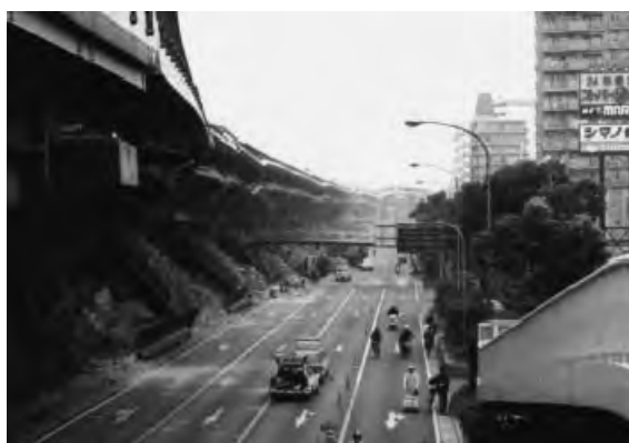
Figure 3: Destructive damage to bridges in 1995 Great Hanshin-Awaji Earthquake (MLIT)
