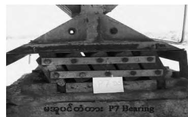
Photo 1: Deformed locker shoes on end pier Photo 2: Deformed shoe on pier 7
