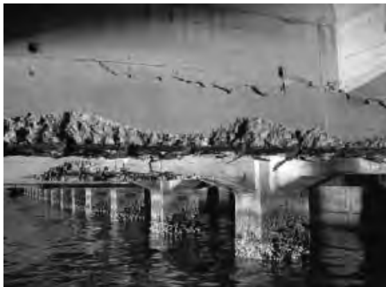
Figure 14: Deteriorated RC wharf due to chloride corrosion (Photo: Dr. Ema Kato)
