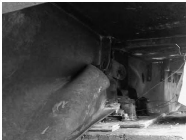
Photo 3: Damaged I- Beam
