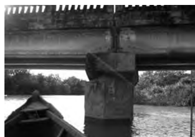
Photo 4: Expansion of bridge seat
