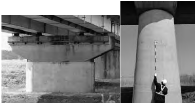
Figure 7: Bridge piers strengthened (left, no damage) and before strengthened (right, damaged) (Photo: PWRI)
