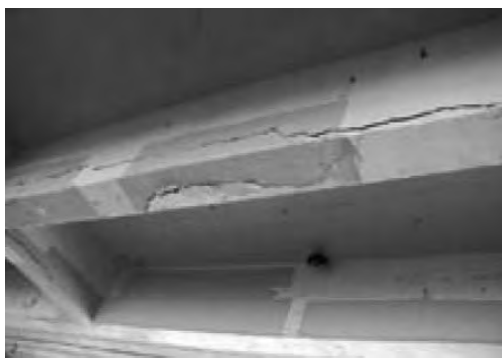
Figure 6: Degradation damage of road bridge main girder (Ministry of Land, Infrastructure and Transport website)
