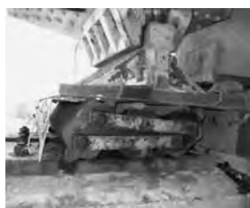
Photo 1: Deformed locker shoes on end pier Photo 2: Deformed shoe on pier 7
