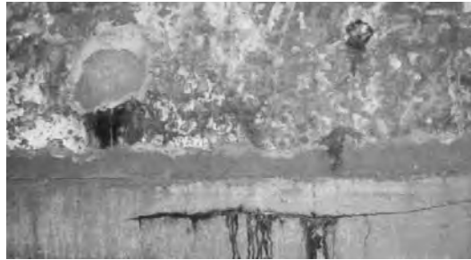
Figure 1: Example of salt damage
