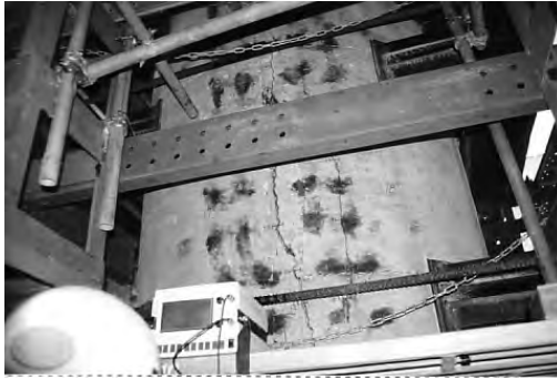
Figure 4: Cracks on highway concrete bridge pier
