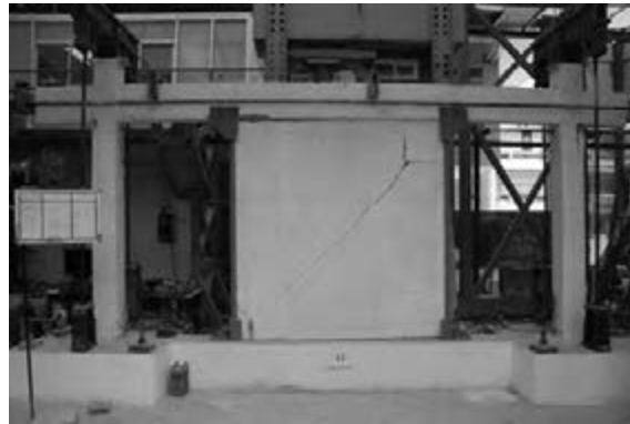
Figure 6: Retrofitted masonry-infilled RC frame (MIRCF04) with the innovative scheme at 2.5% drift (test terminated for safety reason)
