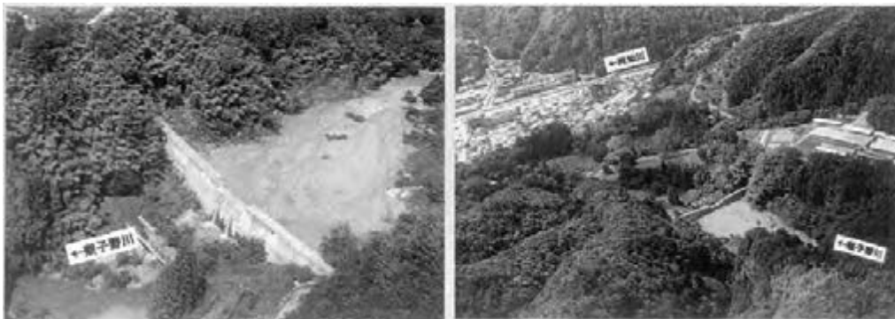
Figure: 13 Original sabo dam of Japan for Nagano city protection
