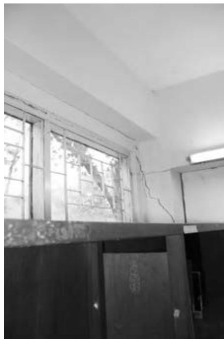
(c) Crack in first floor (viewed from inside)
