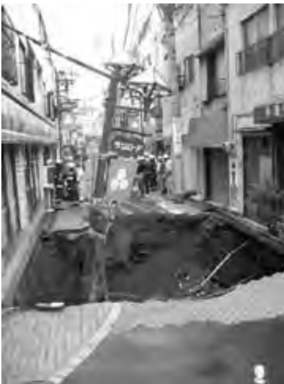
Figure 1: Cave-in accident (6 th August, Tokyo Newspaper)
