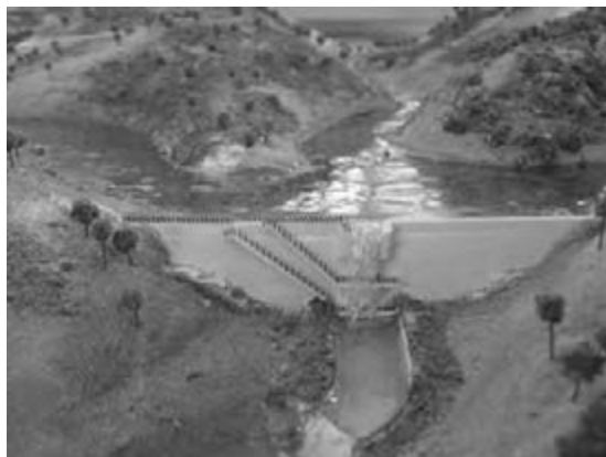
Figure 14: Sediment–water storage dam No.2 of Mae–Ngon basin
