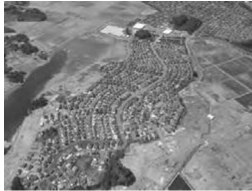
Figure 4: Houses located on a hilltop which were spared tsunami damage
