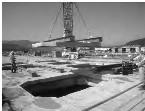
Figure 2: Sampling of a slab
