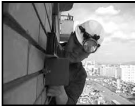
Figure 3: GSR-24 is being placed outside of the building
