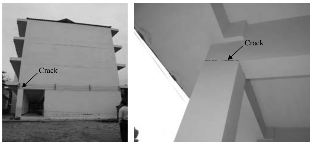
(a) Side view (b) Crack at upper end of the first floor column
