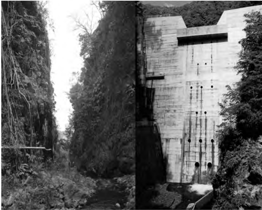
Figure 12: Similarity of Sediment – water storage dam site No.1 (Left) and original sabo dam (Right)
