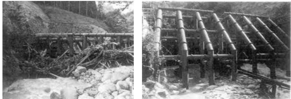
Figure 15: Original slit sabo dam of Japan
