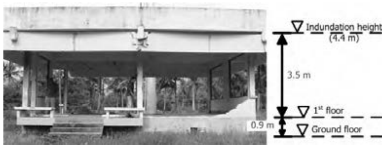
Figure 1: The former office of Thai Meteorological Department in Phang-Nga (Lukkunaprasit et al., 2008)
