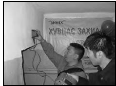
Figure 4: Profometer-5 indicating reinforcing bars
