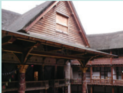
Shakespeare Globe Theater, London, Britain Reconstruction of historical architecture In general, thatched roof is not permitted in down town area, but this architecture permitted by using fire resistive board and a sprinkler system in the roof.
