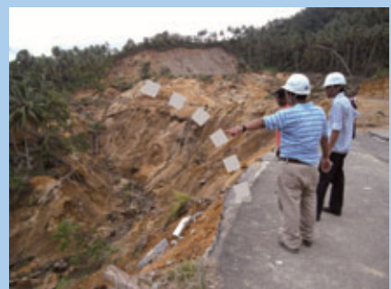
Large slope failure of volcanic sediment
