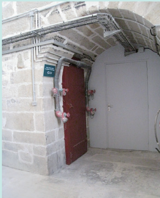
Cathedral Saint Corentin , Quimper, France This stand pipe is the special fire prevention equipment for the wooden roof frame of this cathedral.
