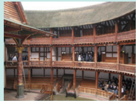
Shakespeare Globe Theater, London, Britain Reconstruction of historical architecture In general, thatched roof is not permitted in down town area, but this architecture permitted by using fire resistive board and a sprinkler system in the roof.
