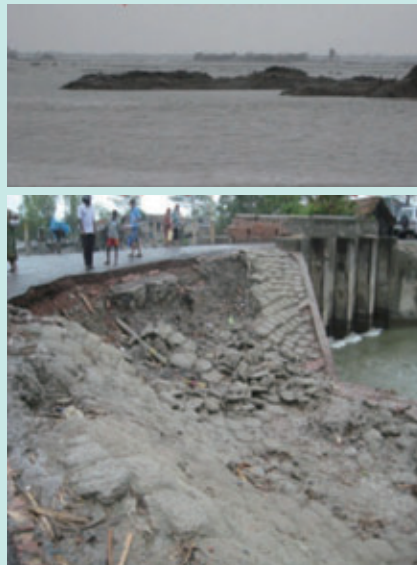
Cyclone Aila damaged embankments at Kapatakha river in Satkhira district.
