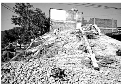
Pancake collapse of building (Abbottabad)
