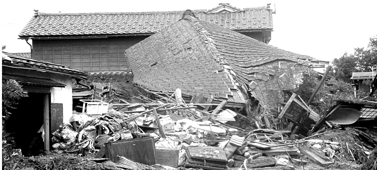
Property damage due to flood caused by failure of embankment
