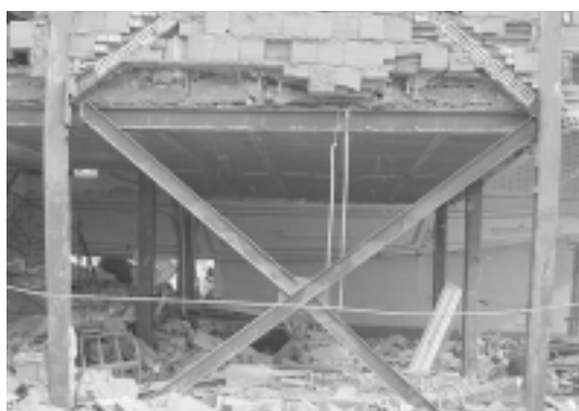
Separation of x-bracing elements from the column due to poor quality of welding
