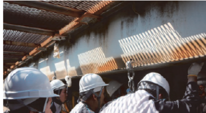
Partially corroded steel girder
