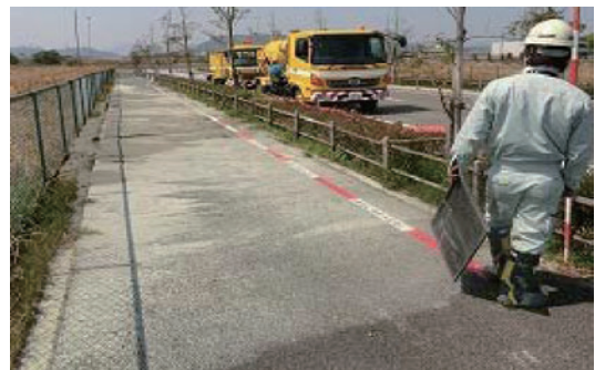
Boiled sand on the side walk and rehabilitation work in Awaji city
