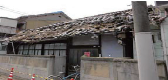
Typical damage to tiled roof in Sumoto city (courtesy Prof. Mikami, Tokushima Univ.)
