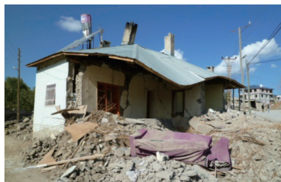
Partially collapsed non-engineered house in Alakoy village, north-east of Van (Nov. 1, 2011)
