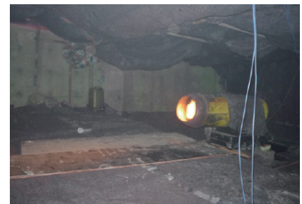
Curing of a concrete slab-on-grade during the winter months using plastic sheets and felt (left) and a diesel heater (right)
