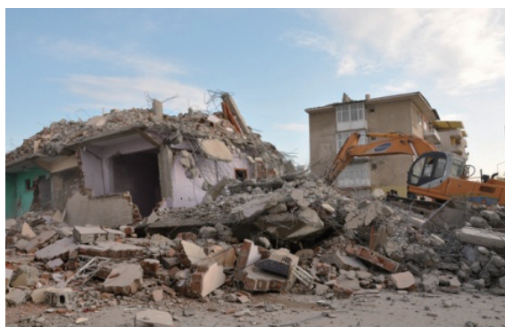
Totally collapsed RC apartment building in the Van city center (Oct. 31, 2011)
