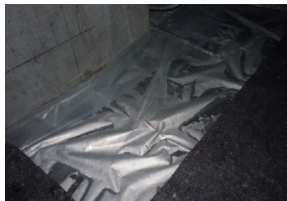
Curing of a concrete slab-on-grade during the winter months using plastic sheets and felt (left) and a diesel heater (right)
