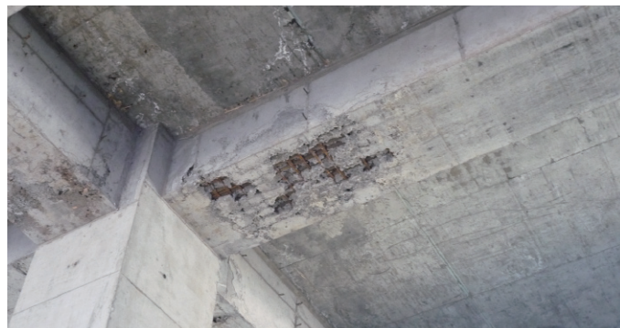
Exposed reinforcement in new construction highlights the importance of improved quality controls
