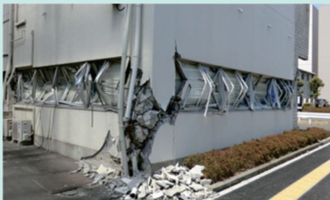
Pancake-type failure of a building in Sendai City, Miyagi Prefecture
