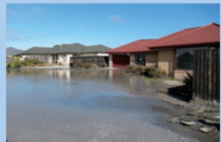
Massive liquefaction at Bexley
