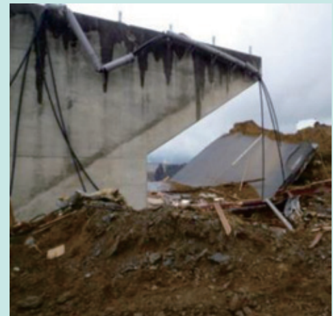
Concrete bridge swept away by the tsunami in Rikuzentakada City, Iwate Prefecture
