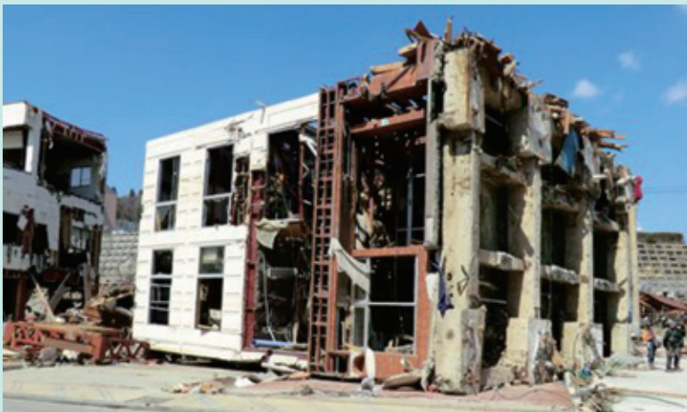
4-story steel building toppled by the tsunami in Onagawa City, Miyagi Prefecture
