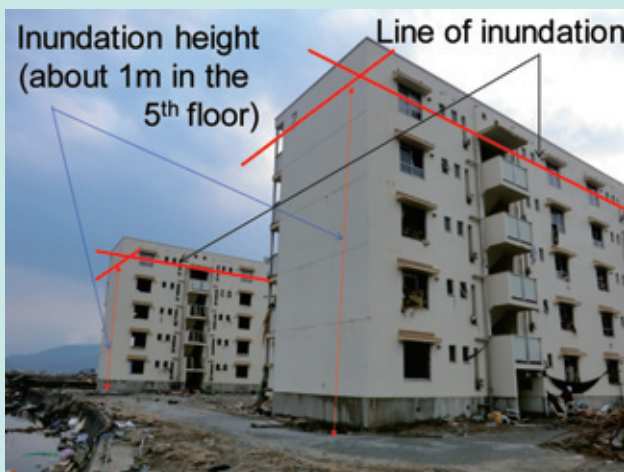
Tsunami damage to 5-story concrete RC apartment building in Rikuzentakada City, Iwate Prefecture
