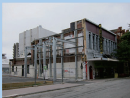
A URM building with temporary shoring survived
