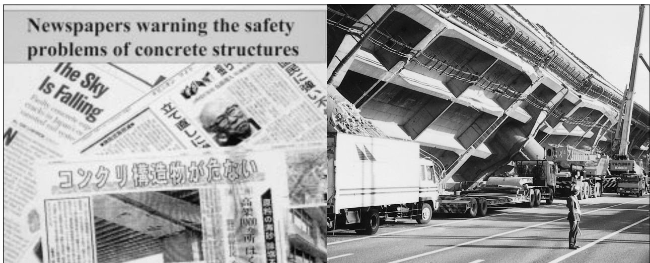
Warning of safety problems of concrete structures in Japan (left) and failure of Hanshin Expressway due to Kobe Earthquake of 1995
