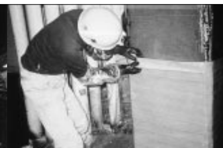
Jacketing of columns with continuous fibre sheets for strengthening structures
