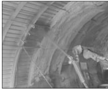
Shotcreting using automated equipment
