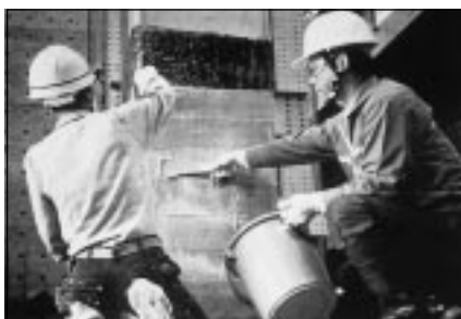
Jacketing of columns with continuous fibre sheets for strengthening structures
