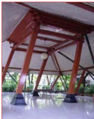
Figure 20 System Joglo the sloping frame building because of earthquake force
