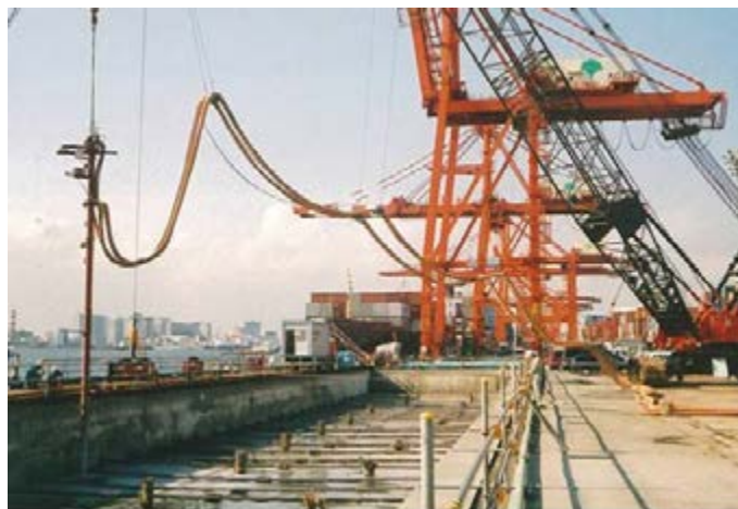
(b) execution of improvement at site
