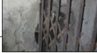
Photograph 12: Blocked emergency stair case in a commercial building are provided improperly and inadequately which poses a threat to the evacuation. In most of the cases escape routes remain blocked (see Photographs 11 and 12).
