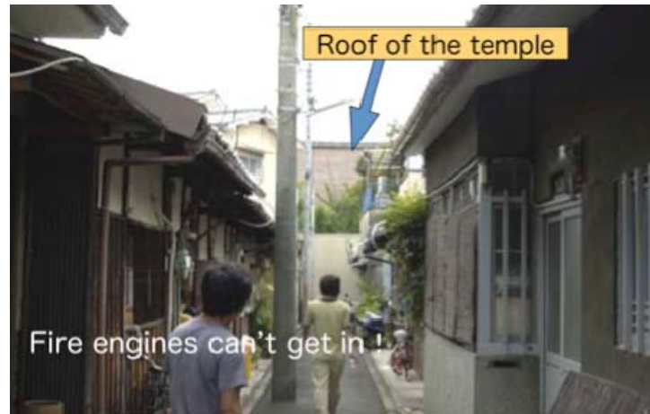
Figure 5 Wooden residential buildings situated closely together in an area containing cultural assets
