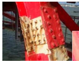
Re-deterioration of repaired part
