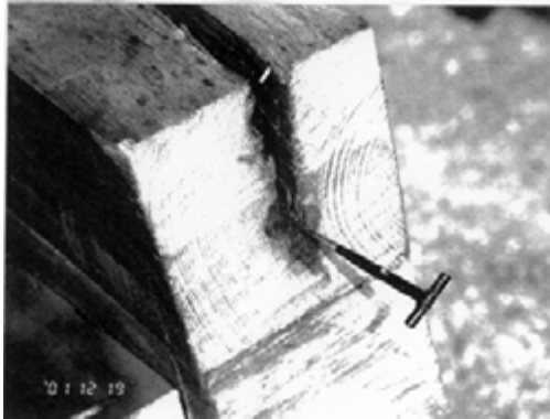
Photo 2: The Decay of the top of “HEIKINGI” (Photo by Kamiyama.)
