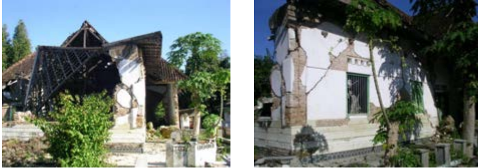
Figure 15 Damage to the house in Bantul, 500m near Opak river
