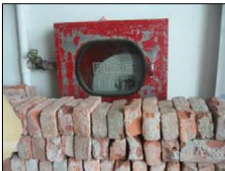
Photograph 7: Blocked hose pipe
