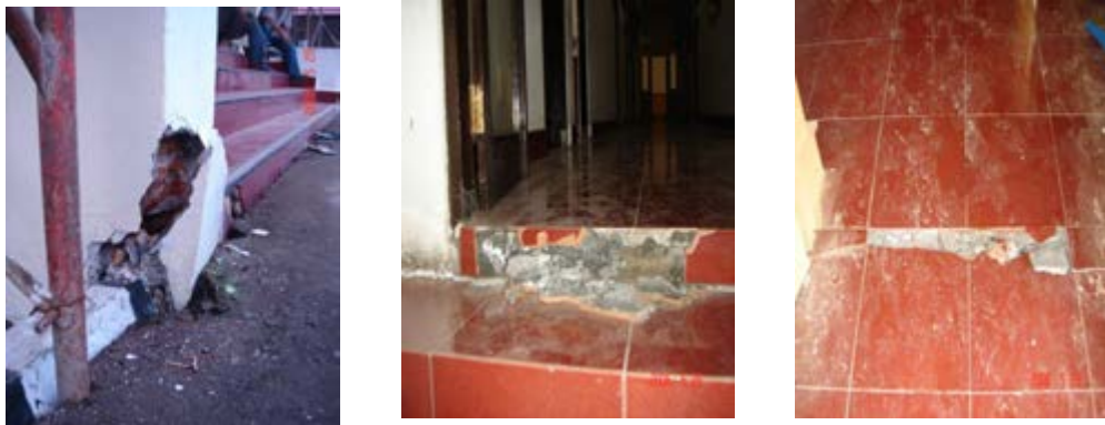
Figure 14 Impact of liquefaction on the building, the city of Yogyakarta
