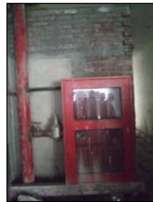
Photograph 6: Hose reel with stand pipe in commercial building
