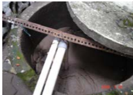
Figure 13 Sand boil, in a home residents, the city of Yogyakarta
