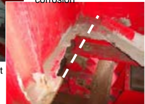
Figure 7: Choshi Oh-hashii Bridge and deterioration of the members
