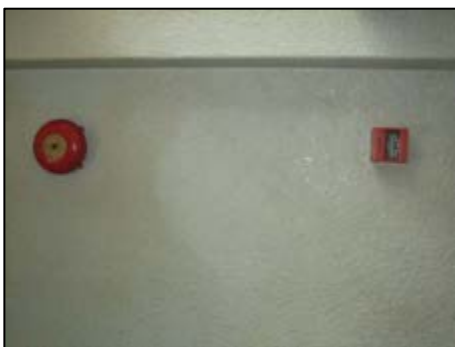
Photograph 9: Fire alarm and fire bell
