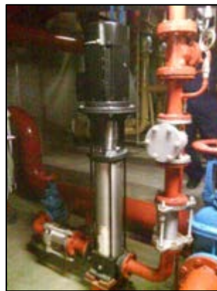
Photograph 5: Jockey pump in commercial building
