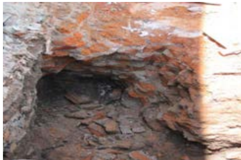
Figure 8 The composition of red brick below the foundation
