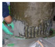
Filled with quick setting mortar
