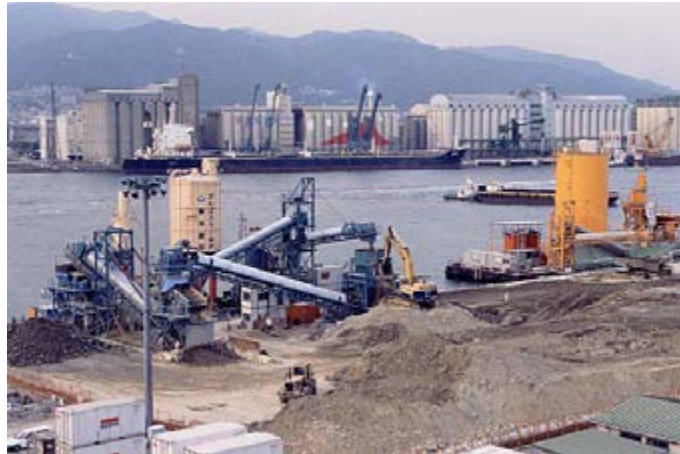
(b) execution of improvement at site Figure 6: Application of Premixing Method at Kobe port
