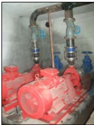
Photograph 4: Fire pump in commercial building
