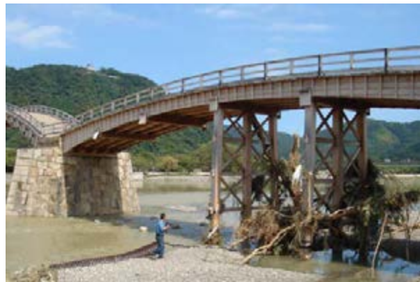
Photo 5: The damage of no.1 bridge after Typhoon
