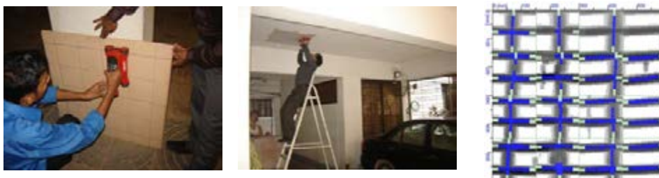
Figure 3(b): Column and slab checking using Ferroskan
