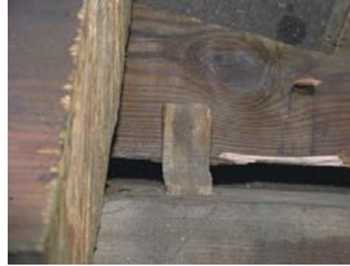
Photo 3: Deformation of dowel between beams
