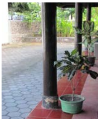
Figure 17 The columns on umpak base
