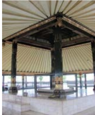
Figure 18 The four columns supporting the Joglo building in the palace of Yogyakarta
