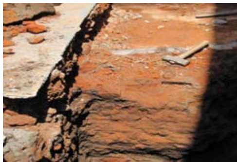
Figure 7 Fractions of red brick as soil stabilization
