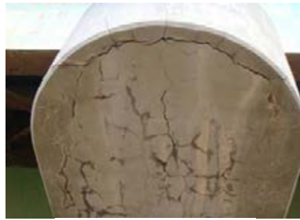
Crack at a pier by ASR
