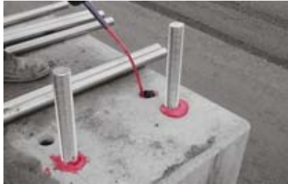
Figure 4: Application of bonded post installed anchorage
