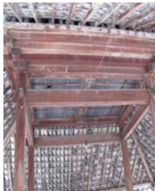
Figure 19 Construction of a fairly stiff tongue connection of beam of the Joglo building
