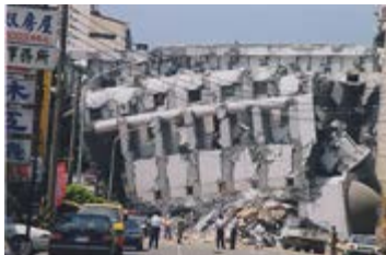
Collapsed condition of XingYiang 向陽 Community
