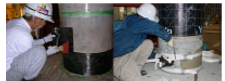
Braced with CFS or polyester bands
