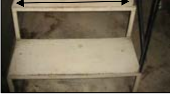
Photograph 11: Narrow emergency stair case in a residential building
